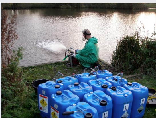
Dosing hydrogen peroxide to raise oxygen levels
