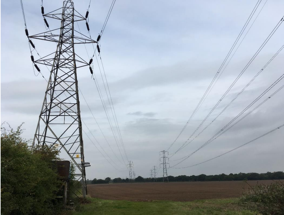
Figure 1: An indicative example of two parallel lines of pylons at Shaw Lane, Kings Bromley
