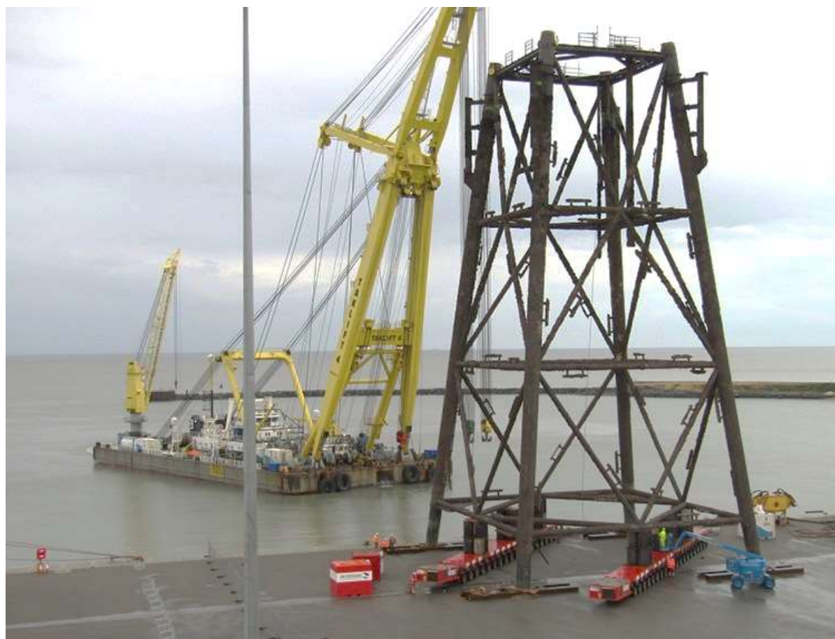
Photo 16 – Moving jacket to decommissioning site (August 2017)
