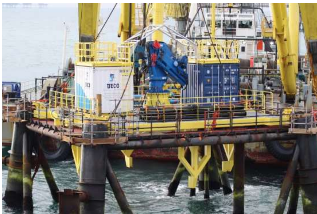
Photo 9 – Installation of rigging platform on Leman BH jacket (July 2017)
