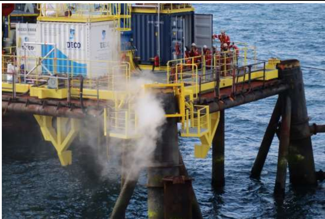
Photo 11 – Cutting holes for the lifting pins (July 2017)
