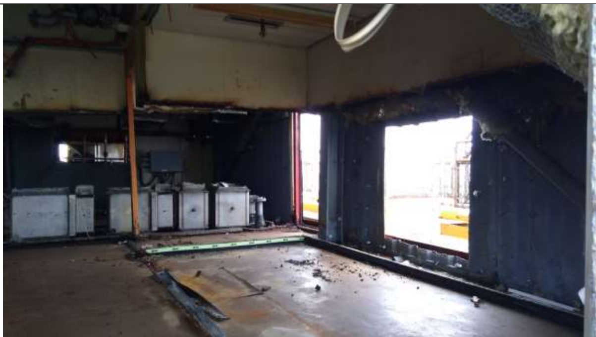
Photo 18 – Soft strip of the topside (August 2017)
