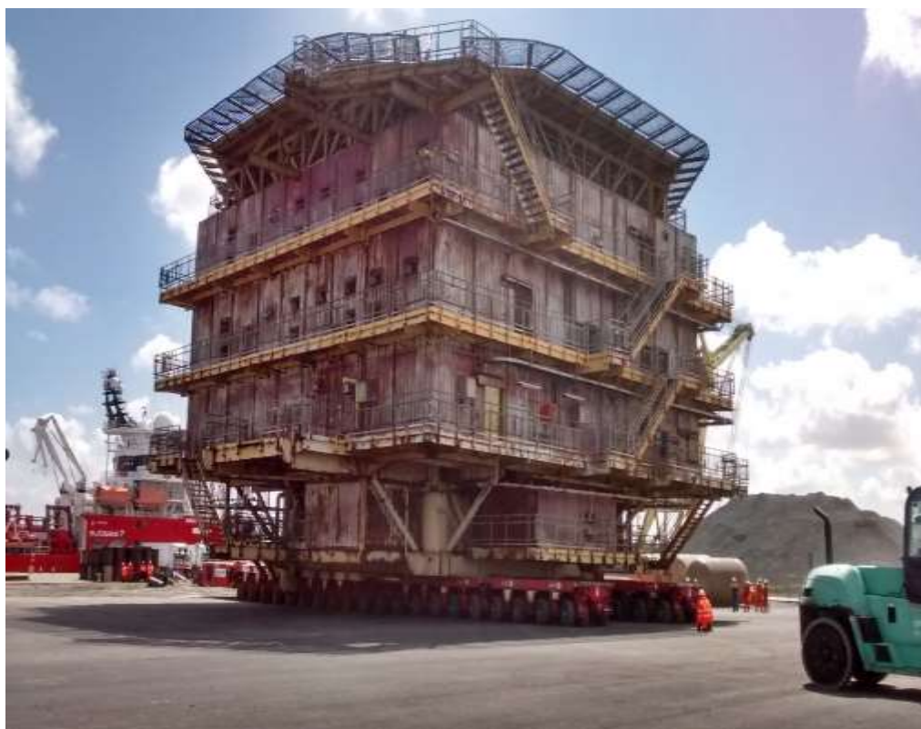
Photo 8 – Transfer of Leman BH topside to decommissioning yard (July 2017)
