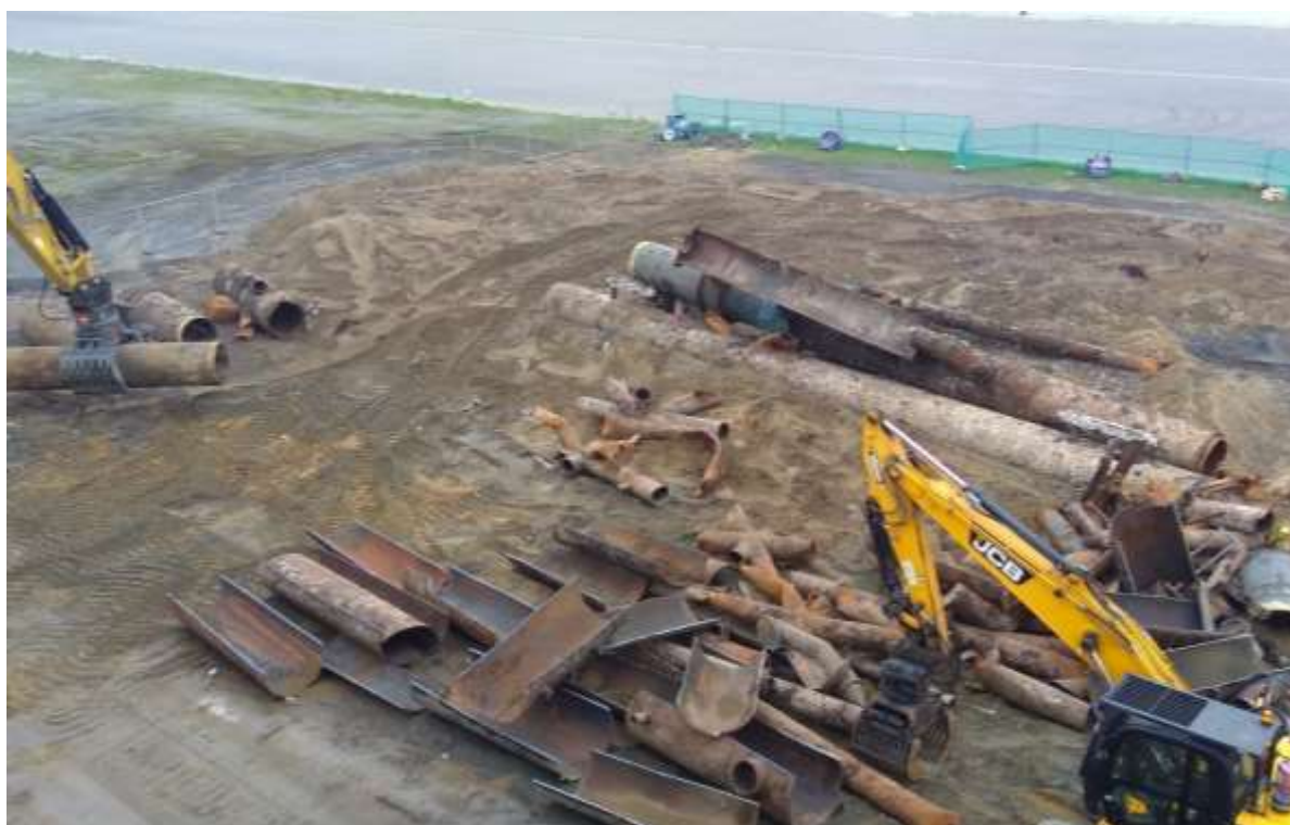
Photo 20 – Jacket Dismantling (September 2017)
