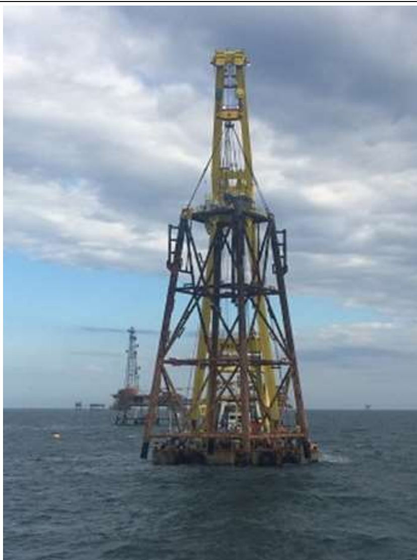
Photo 14 – Lifting of jacket (August 2017)
