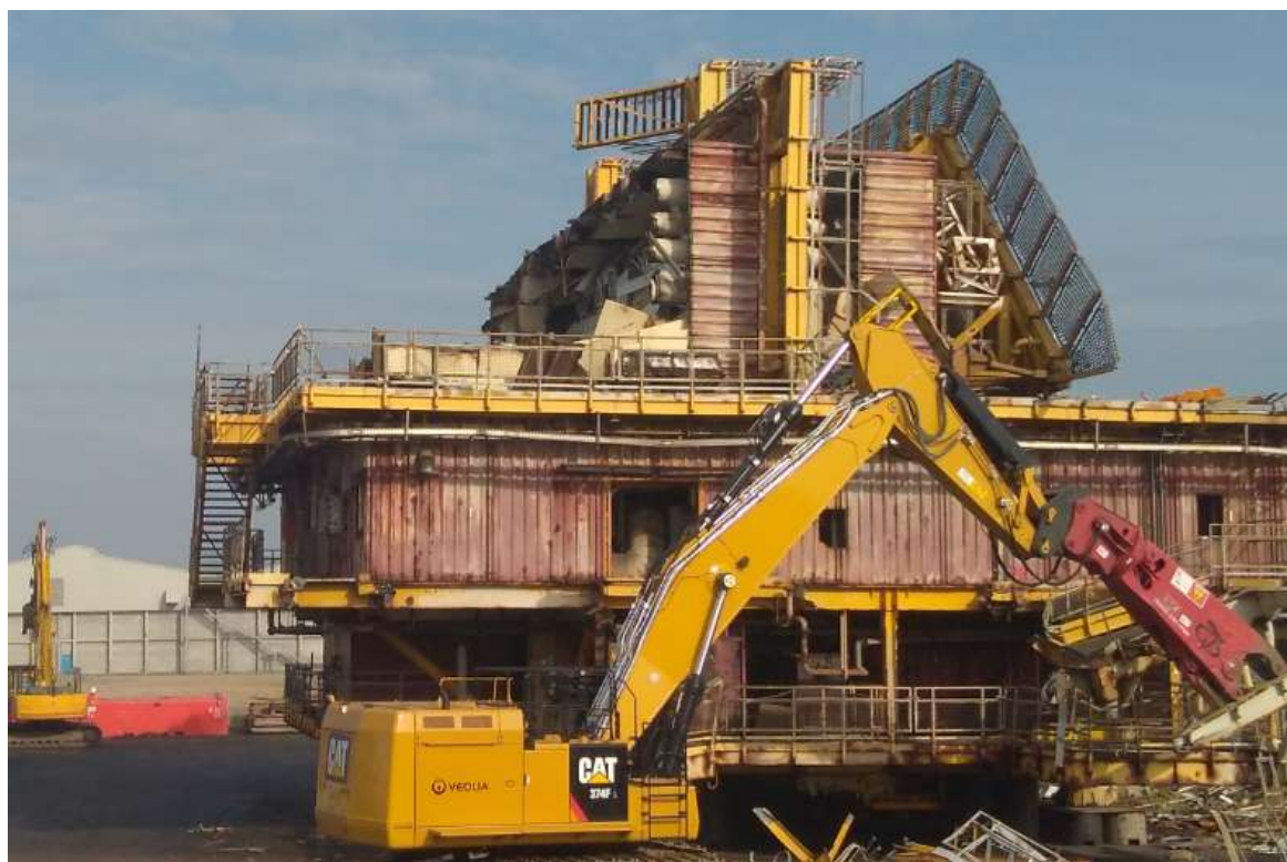
Photo 23 – Topside dismantling (November 2017)
