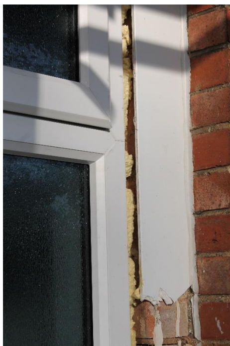
Figure E6 – uninsulated reveal
