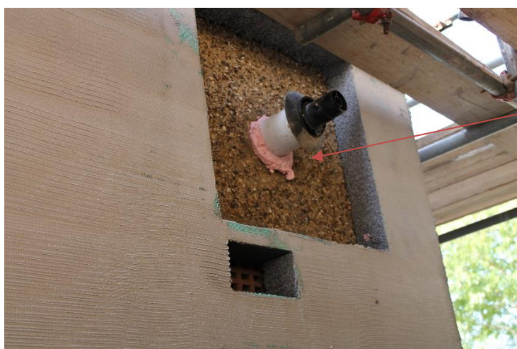
Figure E33 - Cold bridge introduced around gas flue
