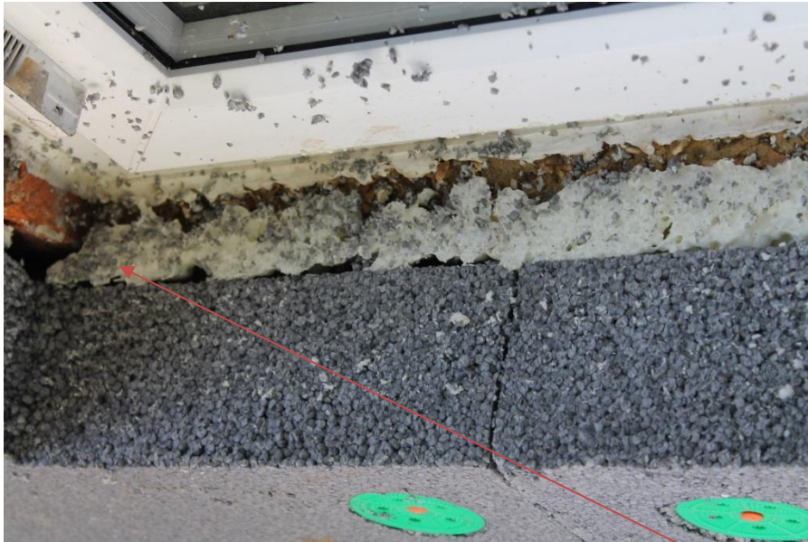
Figure E27 - Cold bridging at window junctions
