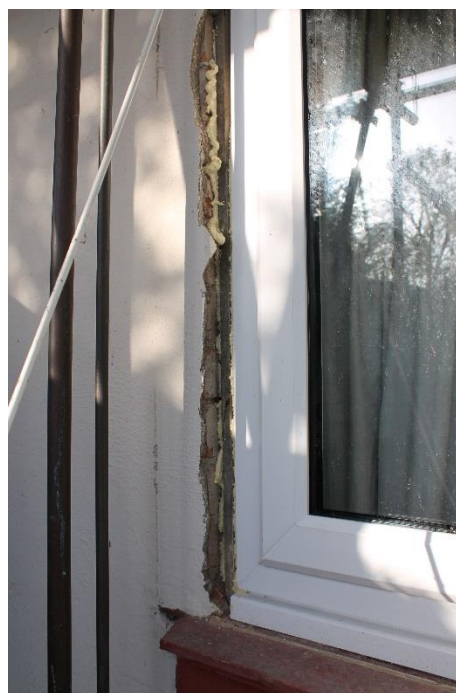
Figure E7 – uninsulated sill
