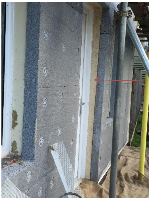
Figure E21 – Cold bridge at door reveal
