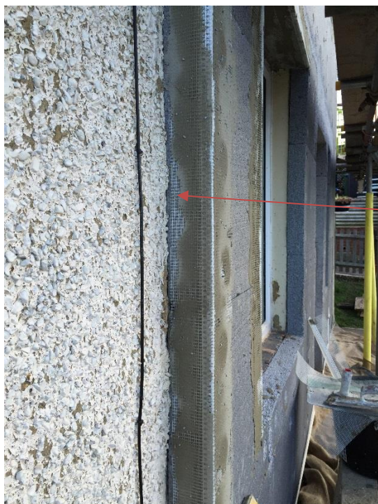
Figure E23 – boundary between insulated and uninsulated dwellings
