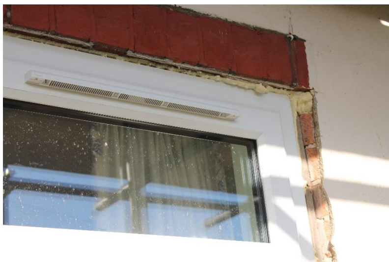
Figure E8 – uninsulated window head
