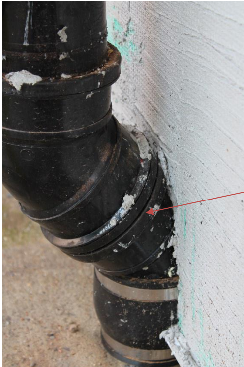
Figure E30 - Soil pipe buried in the insulation
