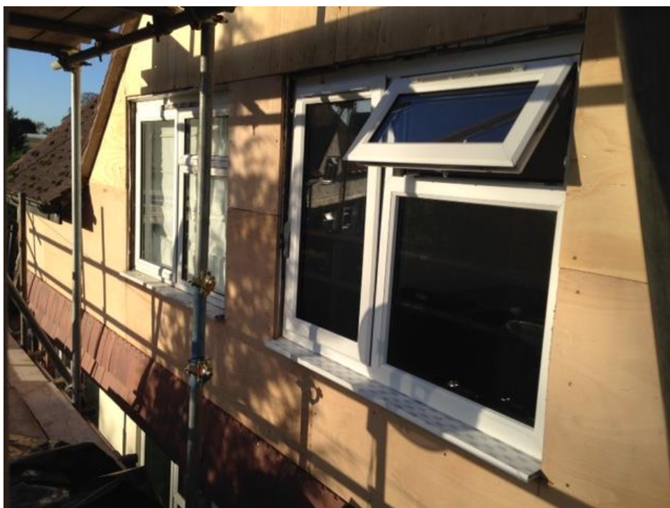
Figure E2 – plywood boarding to timber frame
