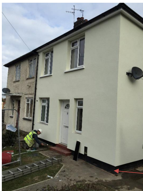
Figure E22 – Cold bridge created by insulation stopped at DPC
