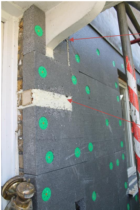
Figure E31 - Canopy not isolated from the building and use of wood as a patten.
