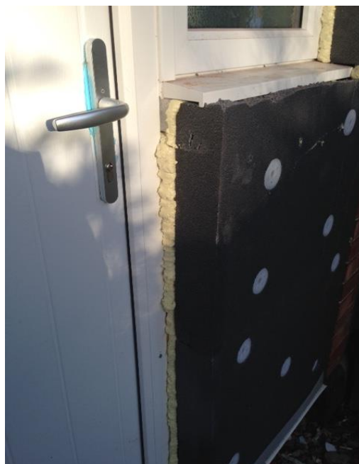
Figure E12- door detail with foam to pack out
