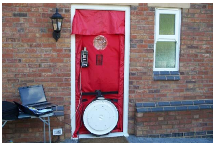
Figure B1 - Air permeability test rig mounted in the front entrance to a dwelling
