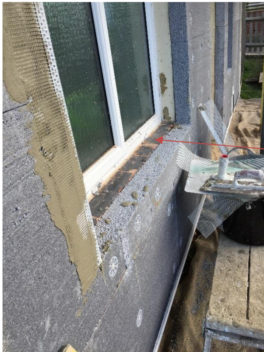
Figure E20 – Cold bridge at window detail
