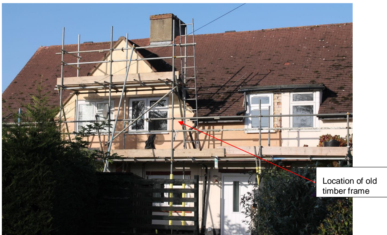
Figure E1 – Front of the dwelling
