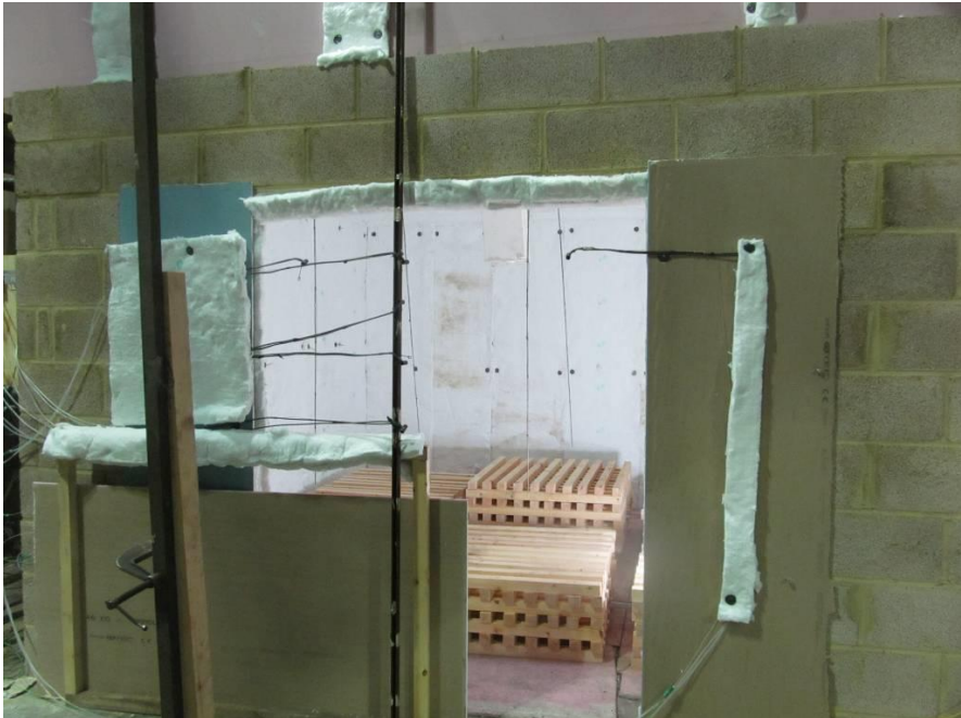
Figure 14 - View of the fire compartment looking in from front ventilation opening
