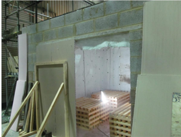
Figure 6 – Front of rig showing cribs before front opening is sealed prior to Experiment 4
