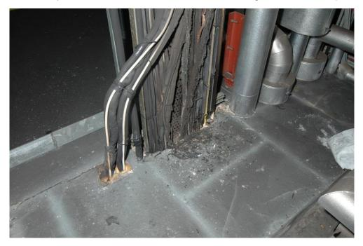
Figure 33 - Effective fire stopping on floor above fire damaged floor
