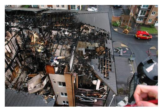
Figure 31 - Partial collapse of development due to extent of fire spread
