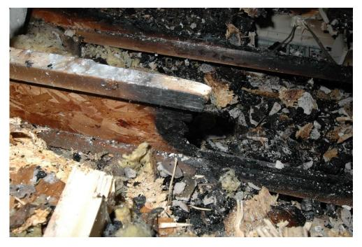
Figure 28 - Damage to engineered floor joists
