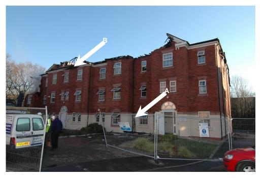
Figure 4 - Arrow A indicates point of fire origin. Arrow B indicates point of break out at roof level
