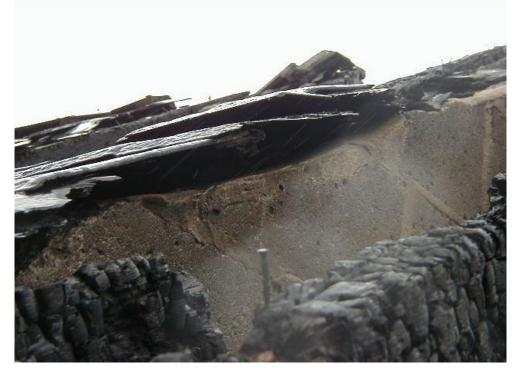
Figure 3 - Lack of fire stopping between compartment wall and roof covering
