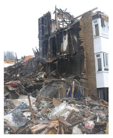
Figure 30 - Structural collapse following fire spread through roof
