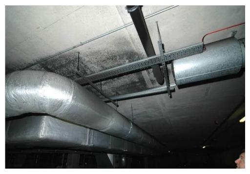
Figure 35 - Flow from impulse jet fan obstructed by HVAC ducting
