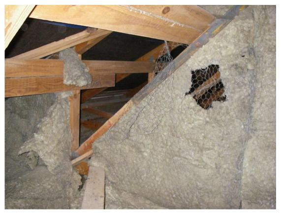
Figure 6 - Fire stopping in poor condition (Image courtesy of London Fire Brigade)
