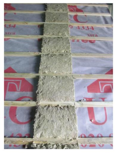
Figure 17 - Insulation between tiling battens prior to fixing roof tiles
