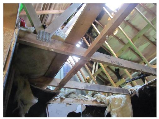
Figure 11 - Undamaged roof trusses above seat of fire
