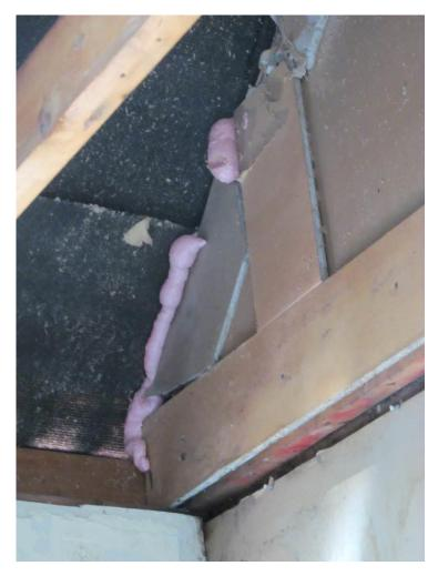
Figure 12 - Sealing between compartment wall and roof construction
