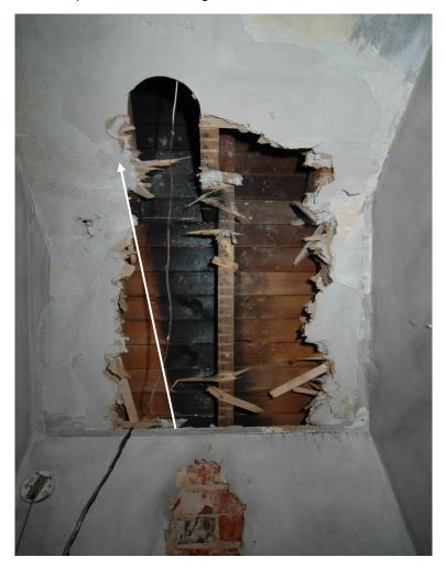
Figure 10 - Close up of fire damage to pitch roof (arrow showing direction of fire spread from wall cavity)
