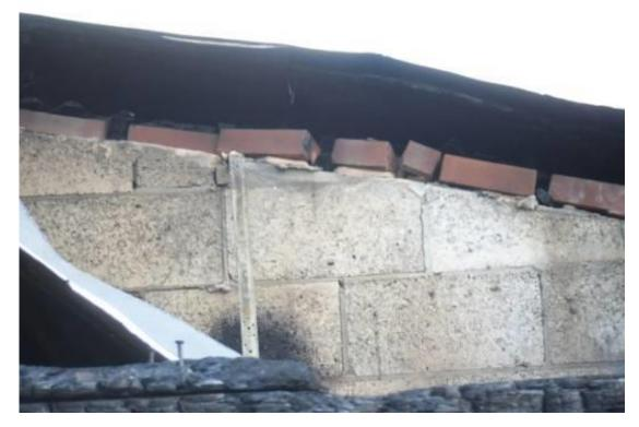
Figure 7 - Attempt to follow roof profile over compartment wall
