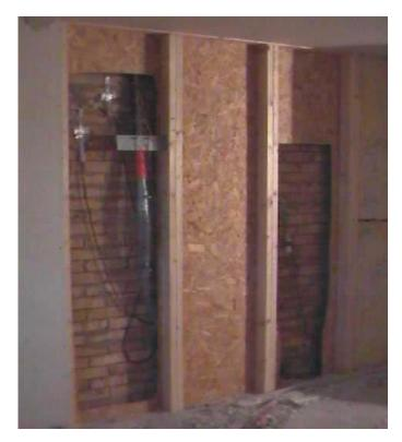
Figure 24 - Internal view of gable end wall with plasterboard linings removed and equipment installed
