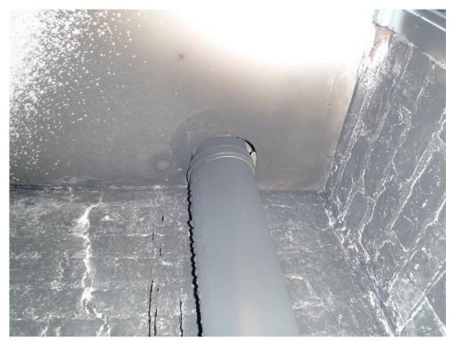
Figure 34 - Inadequate fire stopping around soil pipe penetrating compartment floor
