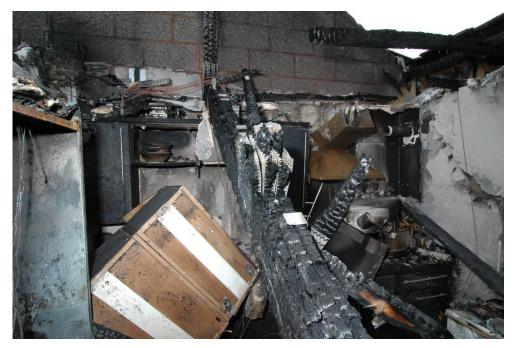
Figure 5 - Roof collapse through ceiling into compartment below
