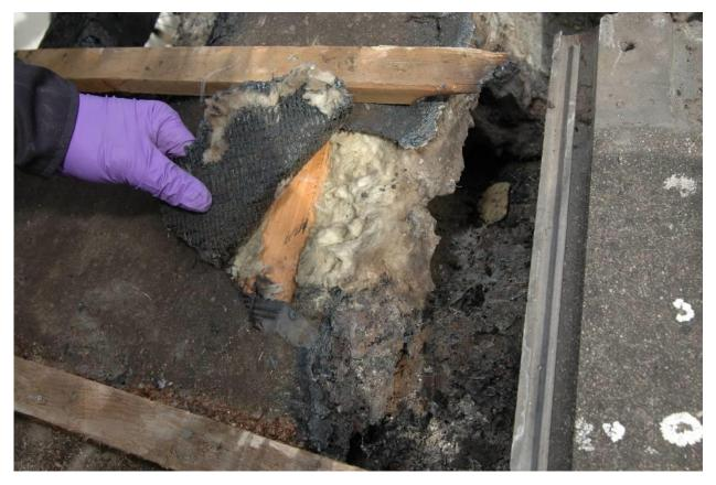
Figure 8 - Fire stopping against underside of sarking felt but not pushed up against underside of roof tiles
