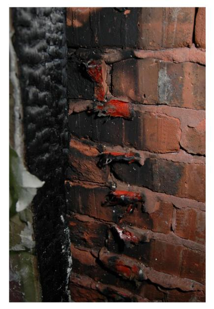
Figure 29 Remains of cavity barrier on external wall
