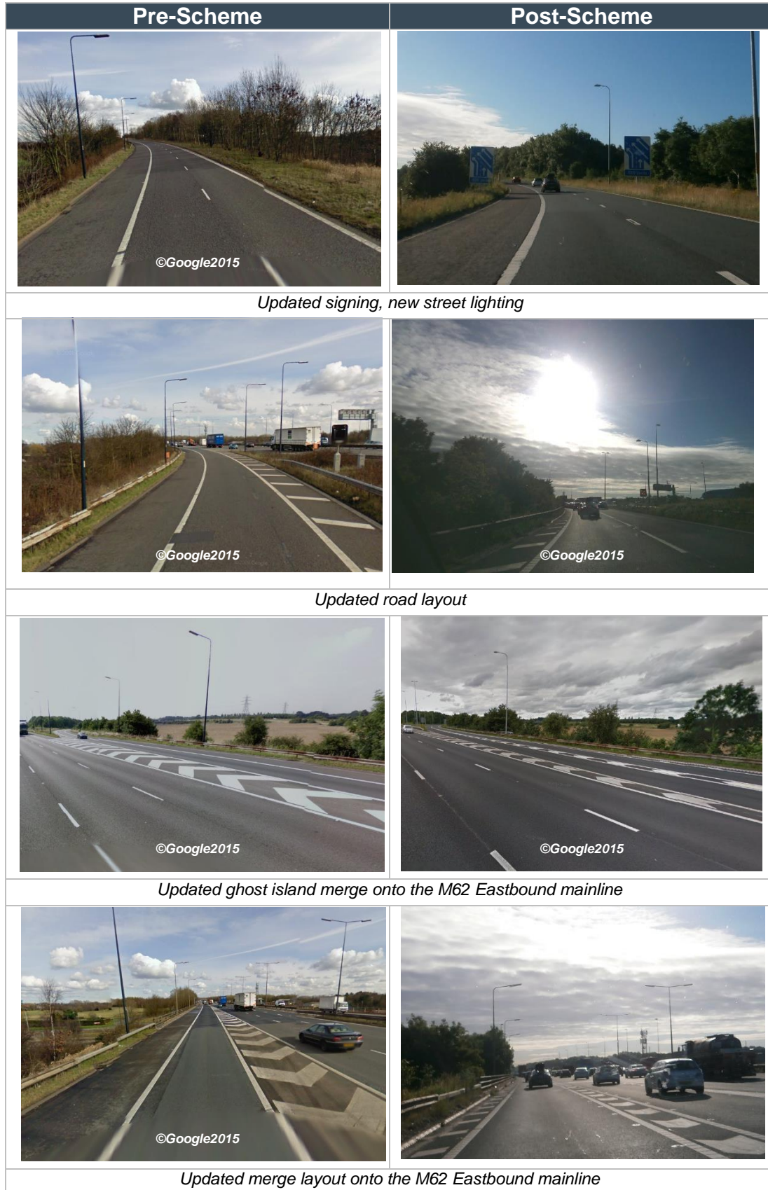
Figure 2.7 – Comparison of Pre- and Post-Scheme Views: M6 Southbound to M62 Eastbound Slip Road
