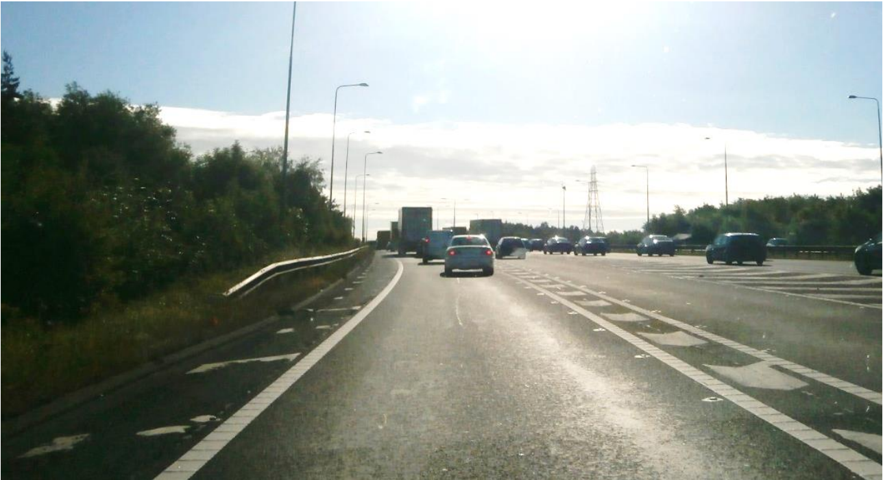
Figure 2.13 – M6 Northbound to M62 Eastbound Slip Road
