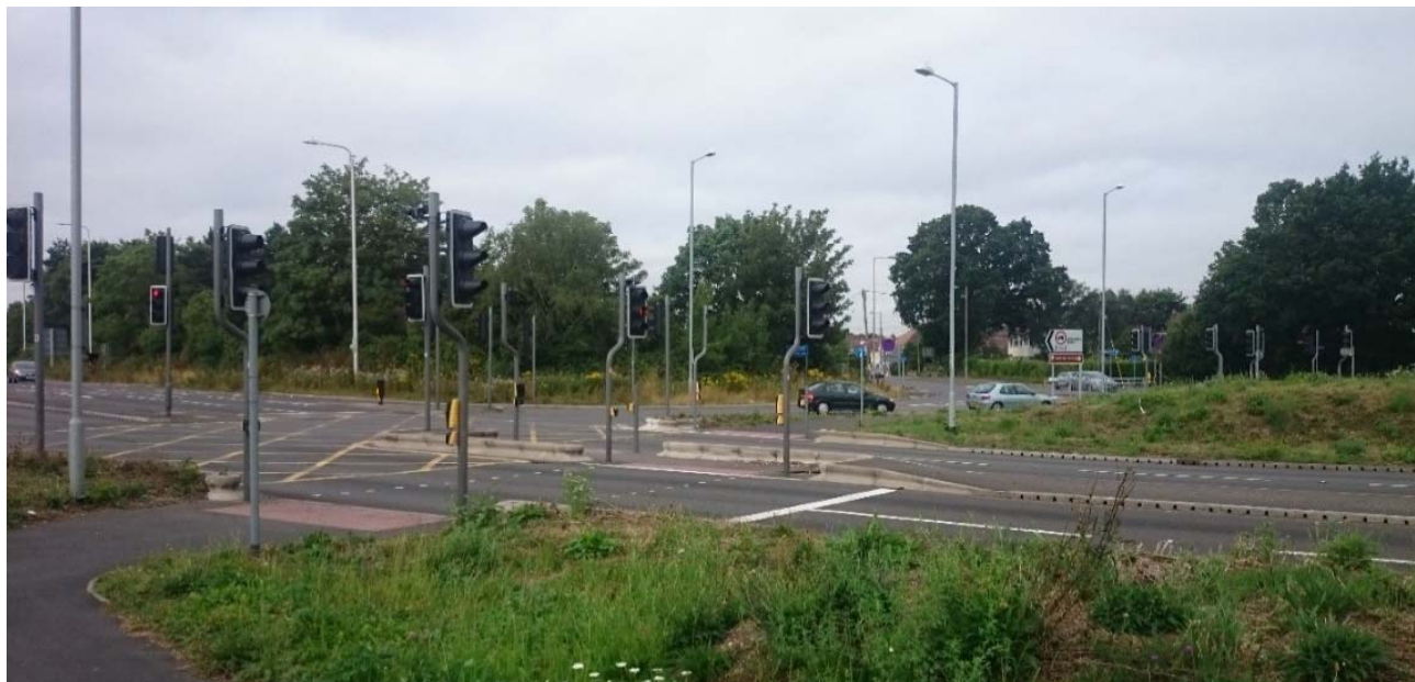
Figure 6.1 – Signals Equipment demonstrating impact on Landscape
