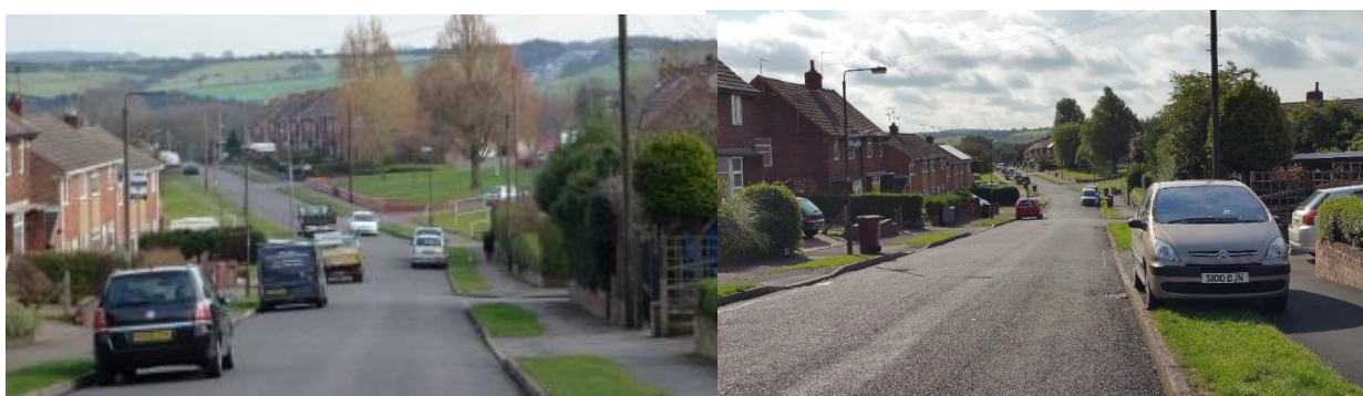
Figure 5-9 Long view of the scheme from Pinxton, with the scheme visible in the background, OYA (left) and FYA (right)
