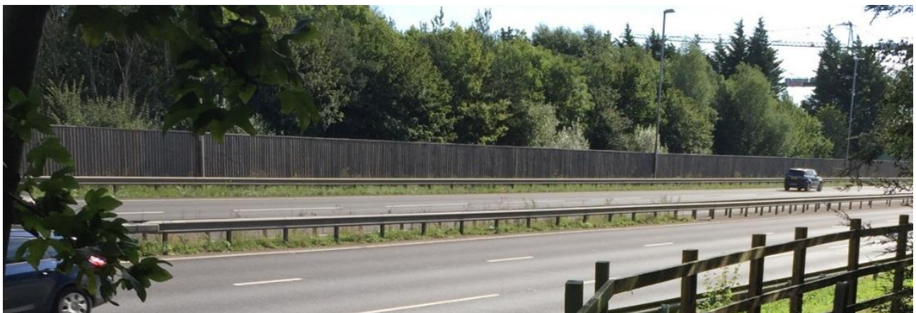
Figure 5-1 Noise barrier on the eastbound carriage from junction 8
