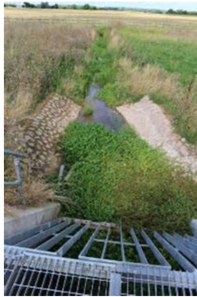
Figure 5.15 (left) Highway drainage ditch at western end of the urban section near Mill Hill roundabout. Figure 5.16 (right) illustrates rural ditch at Pond M with some vegetation clearance required to maintain free flow at the culvert entrance.
