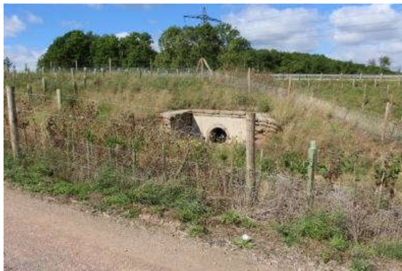
Figure 5.13 Illustrates wildlife underpass WU2 which appears to exit into a fenced planting plot
