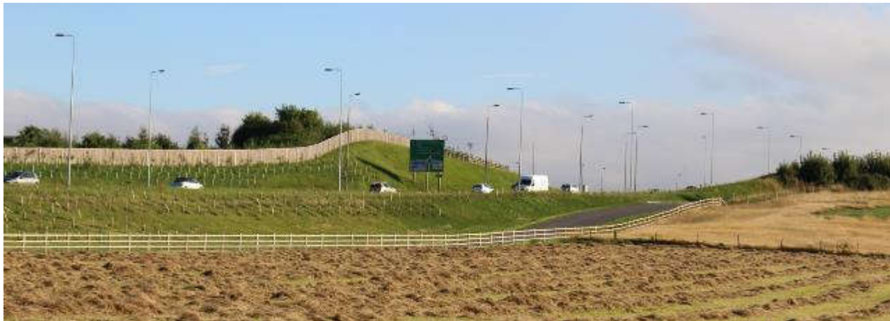
Figure 5.4 view from Fox Covert Lane towards Mill Hill roundabout with acoustic barrier located on top of the cutting earthworks. As built plans indicate that it is a 2.0m high fence on earthworks.
