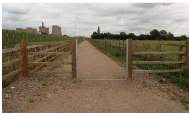
Figure 5.31 example of access point left as gap rather than installing gates along the NMU route.
