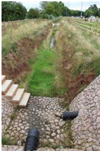
Figure 5.15 (left) Highway drainage ditch at western end of the urban section near Mill Hill roundabout. Figure 5.16 (right) illustrates rural ditch at Pond M with some vegetation clearance required to maintain free flow at the culvert entrance.
