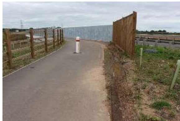
Figure 5.29 (left) Bollard retrofitted presumably to restrict unauthorised vehicle use on the NMU route.
