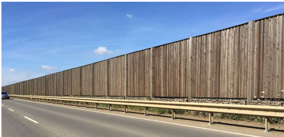
Figure 5-2 Noise barrier east of Marston Junction
