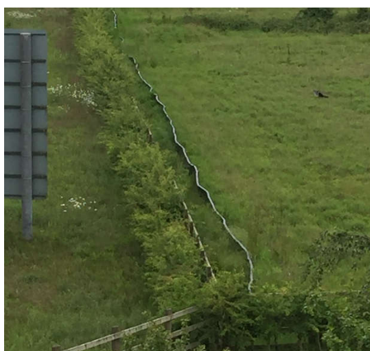
Figure 5-16 Example of amphibian-proof fencing located along the A421
