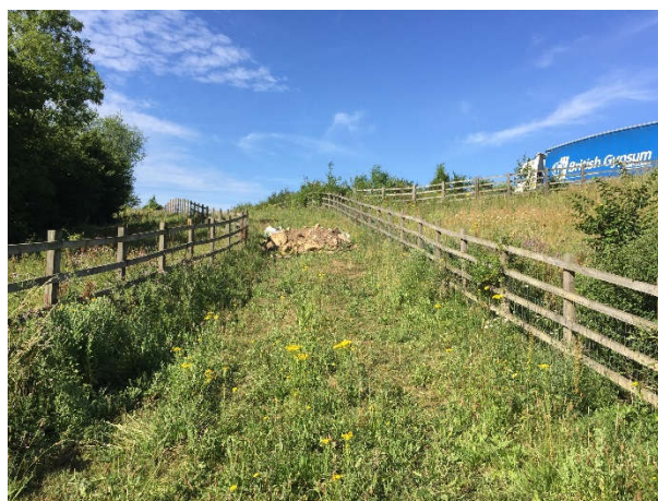
Figure 5-25 Bridleway near North Common Farm underpass blocked with rubble
