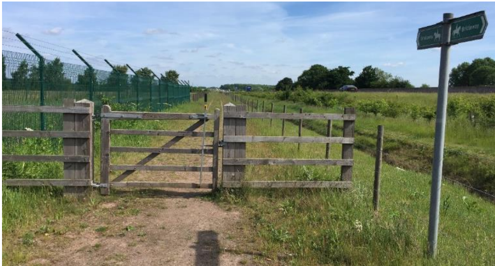
Figure 5-22 Saxondale Bridleway Overbridge
