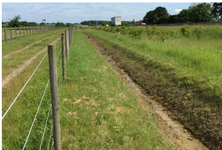
Figure 5-17 Drainage ditch north of Roehoe junction
