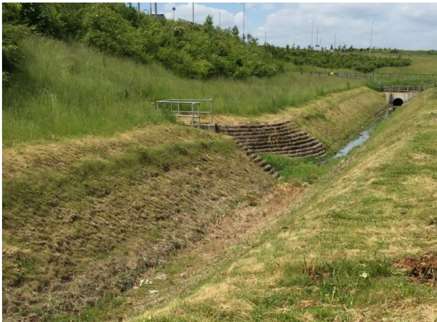
Figure 5-18 Ditch leading to pond 8 and 9
