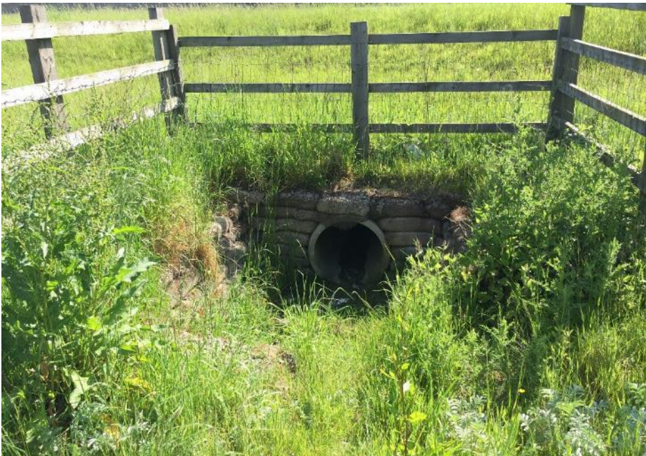
Mammal tunnel BT01
