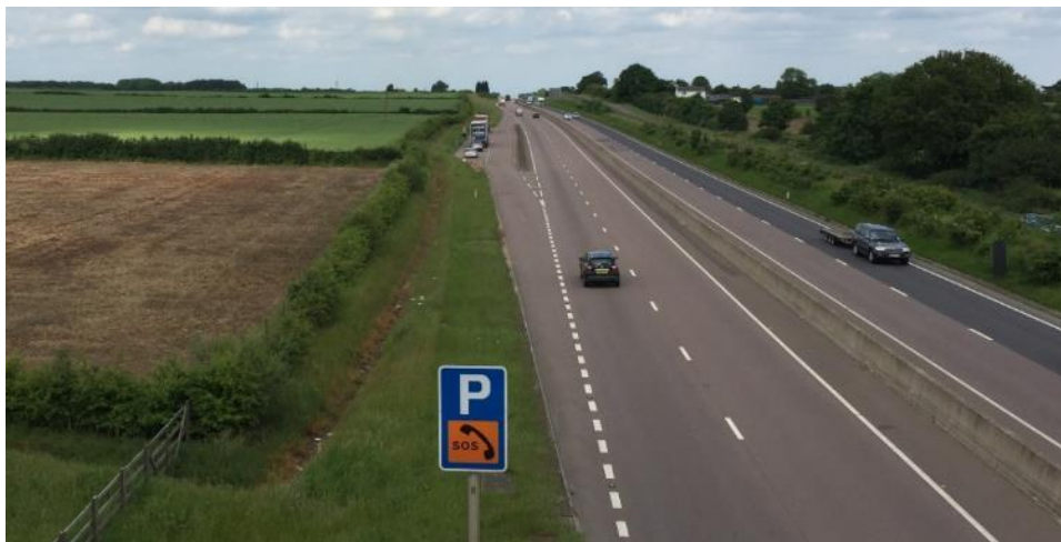
Figure 5-26 Lay-By north east of Car Colston Overbridge
