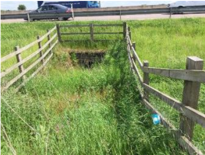
Mammal tunnel BT14
