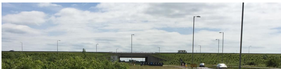
Figure 5-5 Lighting within Stragglethorpe junction
