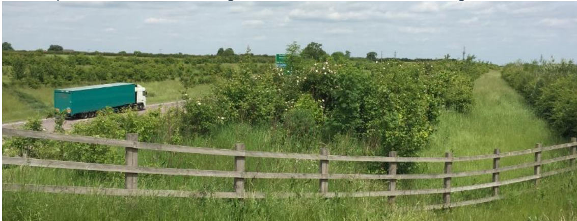
Planting west of Saxondale overbridge
