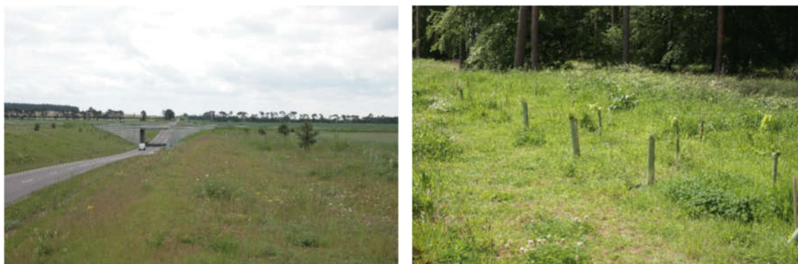
Left: earthworks around structures exhibit smooth, naturalistic flowing contours as expected, and right: woodland edges have been provided.
