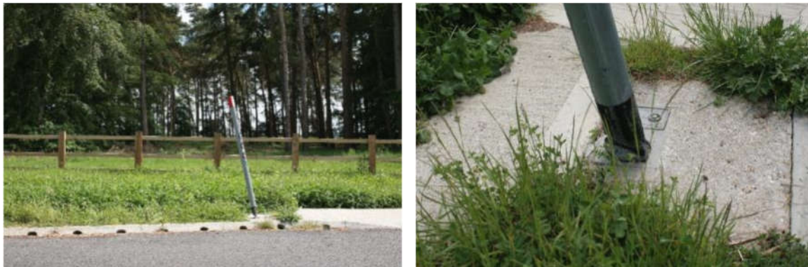
Figure 5-17 Hazard Reflector Post
