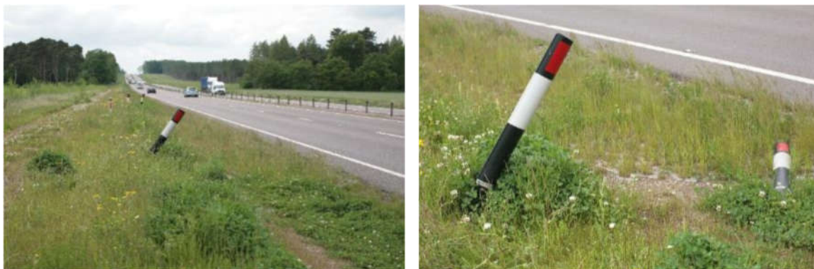
Figure 5-18 Hazard Reflector Posts
