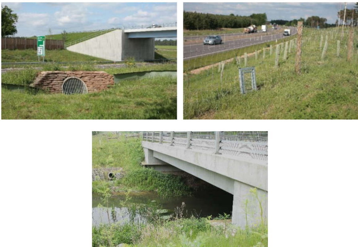
Upper Left: reptile exclusion fencing and underpasses, upper right: one-way mammal gates set within mammal exclusion fencing, and lower centre: mammal ledges at the River Lark cut-off channel.
