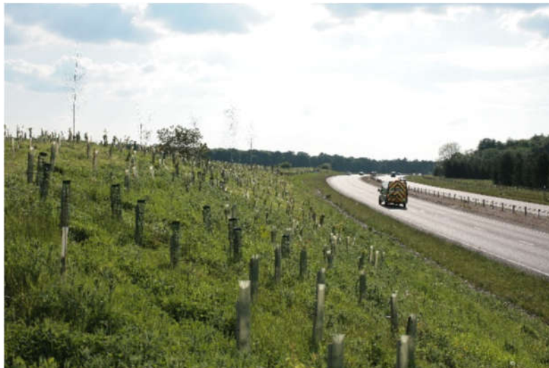
Figure 5-3 Mitigation at Elveden Gap
