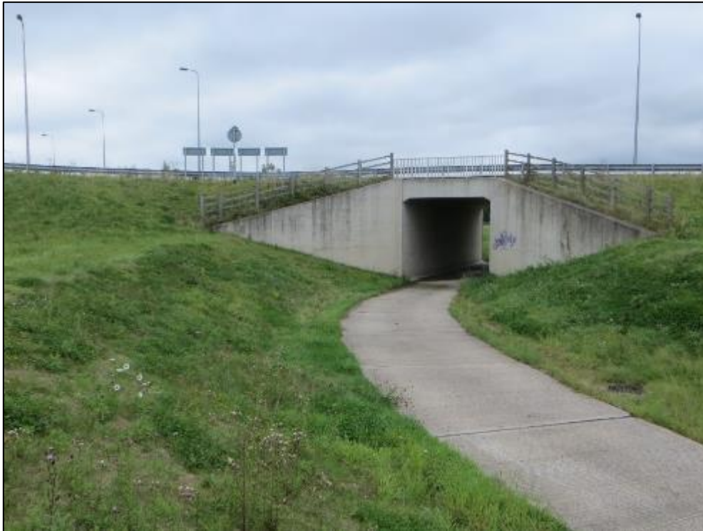
Figure 3-6 New Footway and Underpass Implemented as Part of the Scheme Measures
