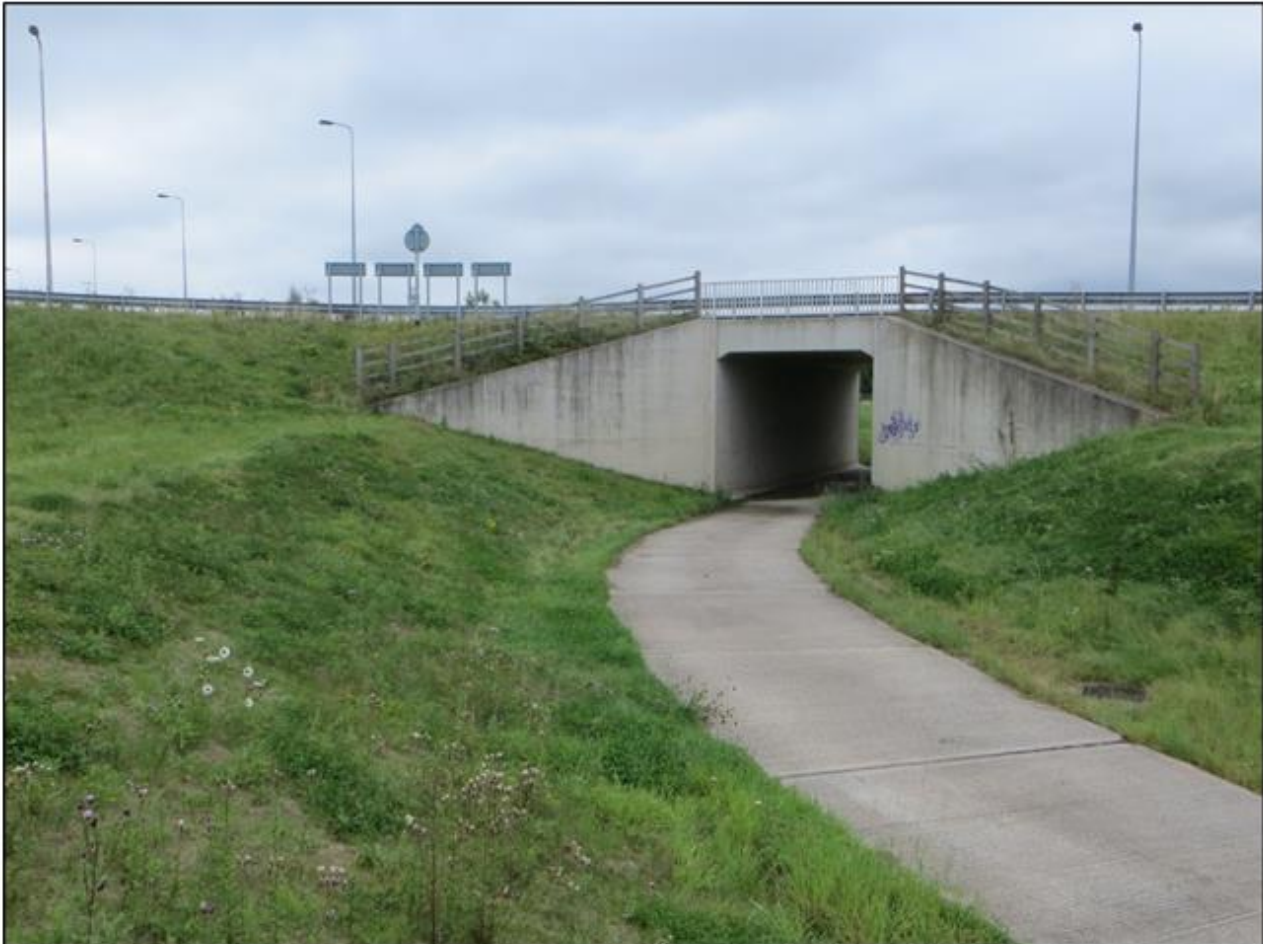
Figure 6-1 New Footway and Underpass Implemented as Part of the Scheme Measures
