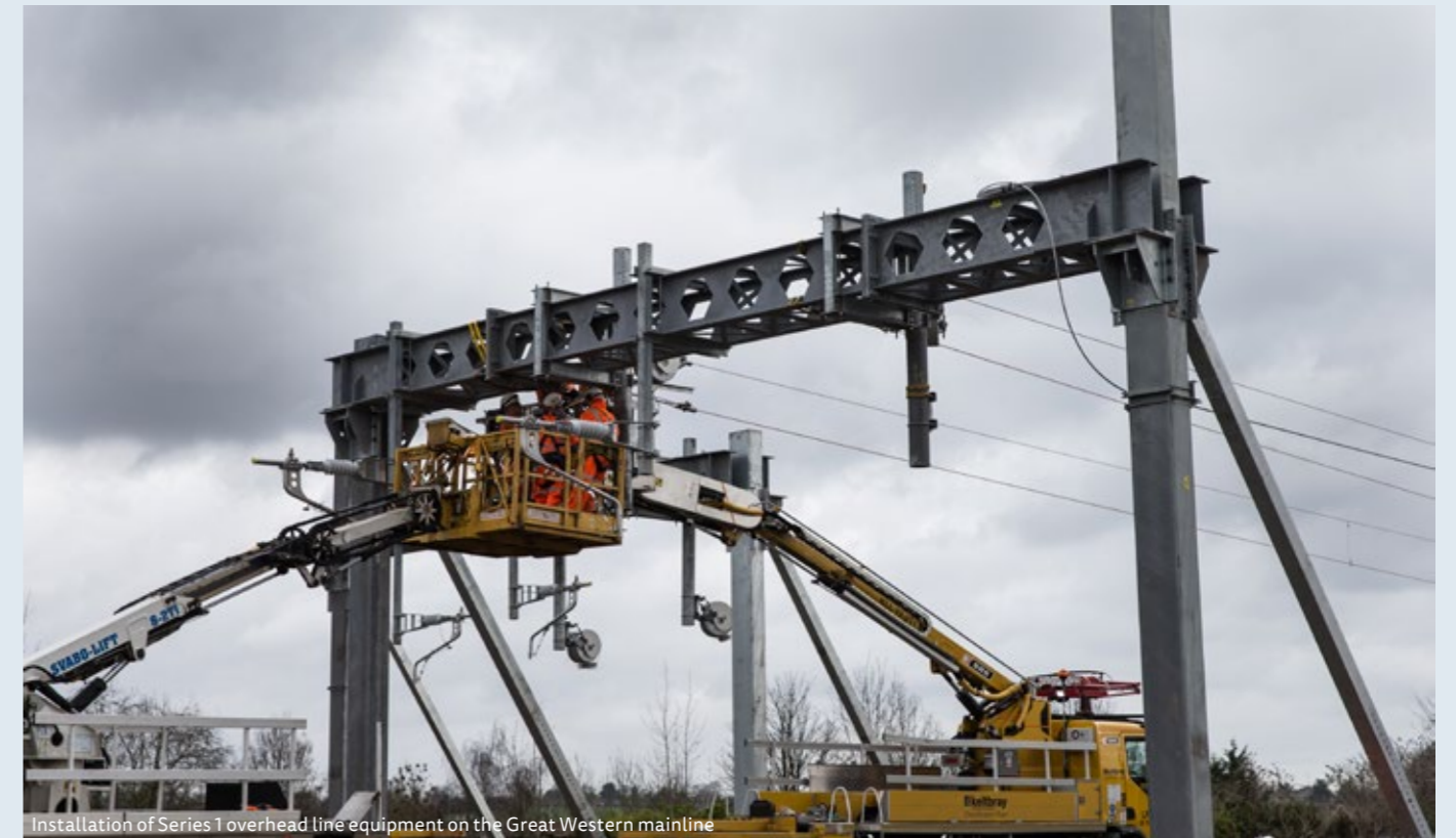
Installation of Series 1 overhead line equipment on the Great Western mainline
