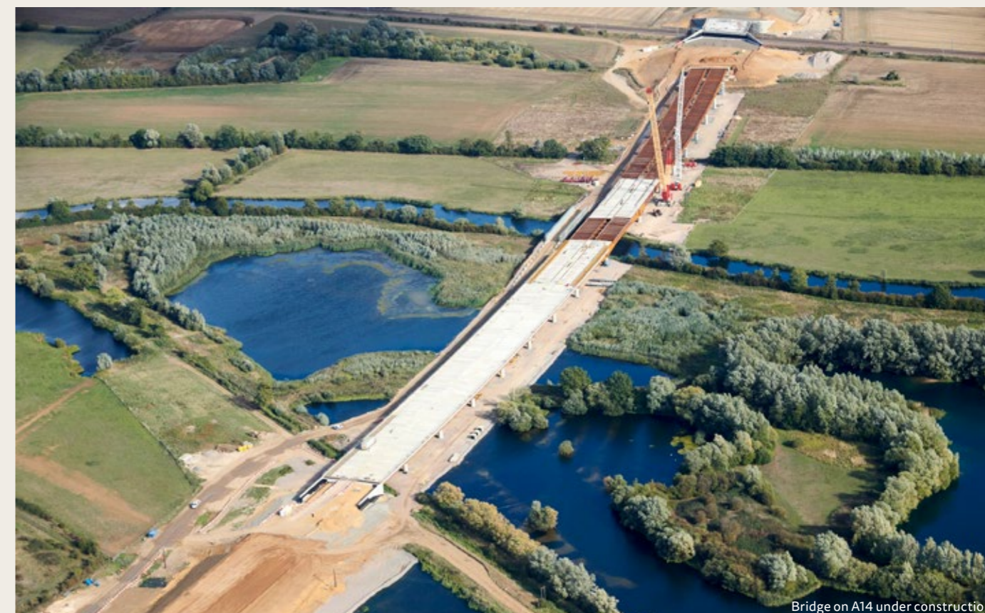
Bridge on A14 under construction
