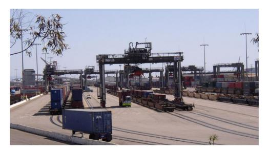
Figure 3: Intermodal ship-to-rail transfer of containerised cargos, port in Long Beach, California<sup>10</sup>
