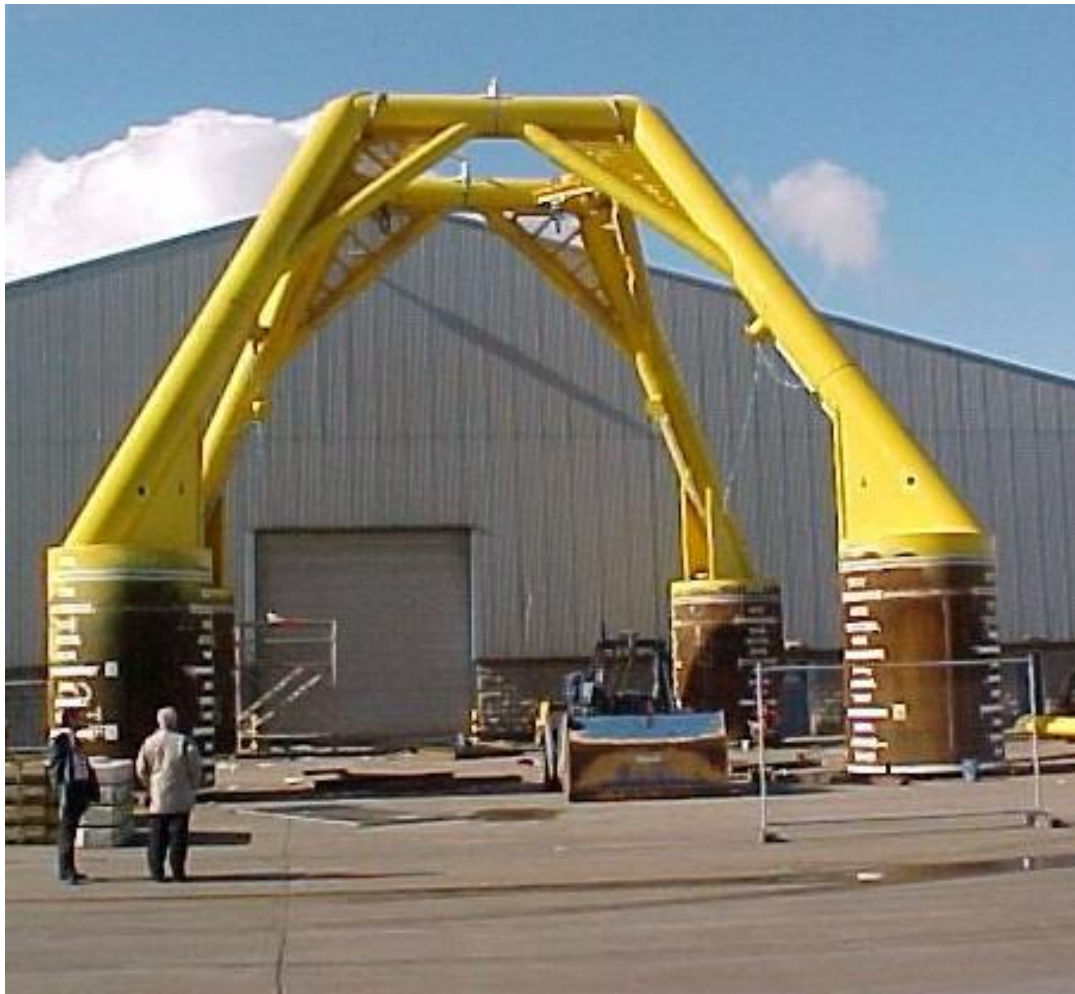
Figure 2.1 Stirling 16/21a-33 Well Head Protection Structure
