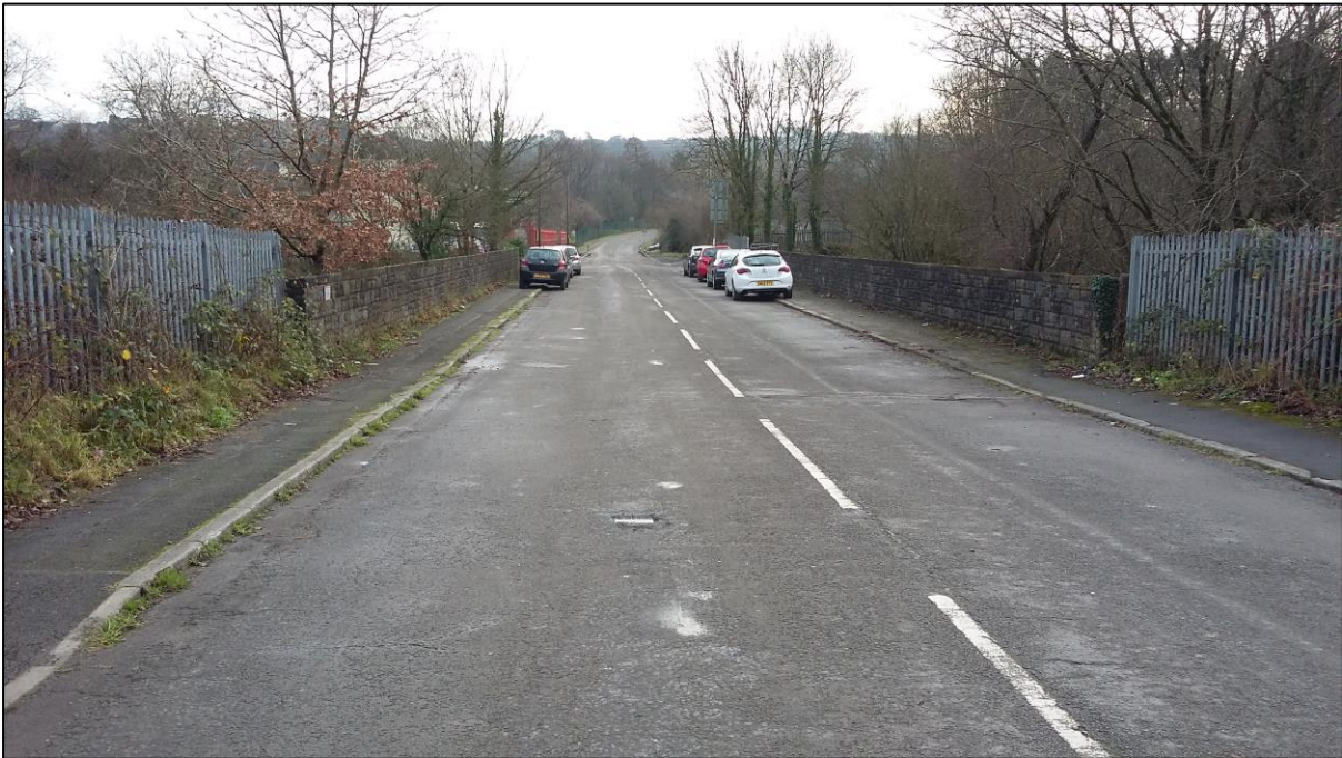
Fig 9d West Wales / Swansea North Parkway approach road via Bryntywod
