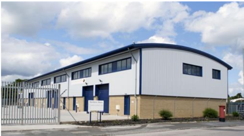
Figure 6.2.3 New CPD units on Dawlish Business Park
