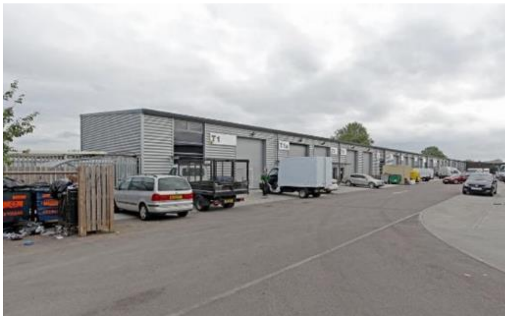
Figure 6.5.7 New CPD units in Leyton Industrial Village
