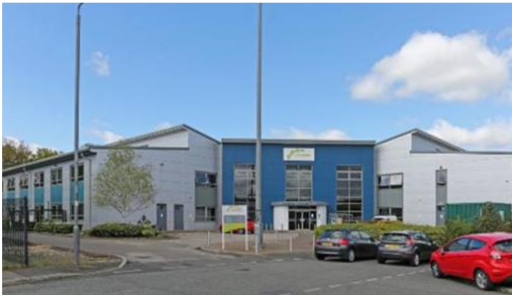
Figure 6.3. 3 New CPD units – Turbine Innovation Centre
