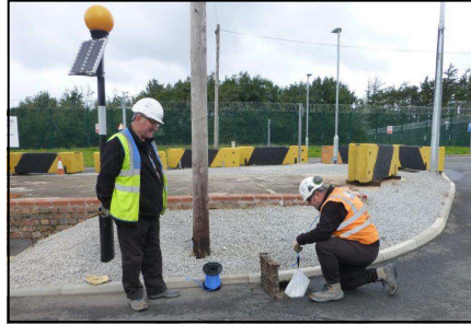
Combating pollution: pillow being applied to a drain on Site
