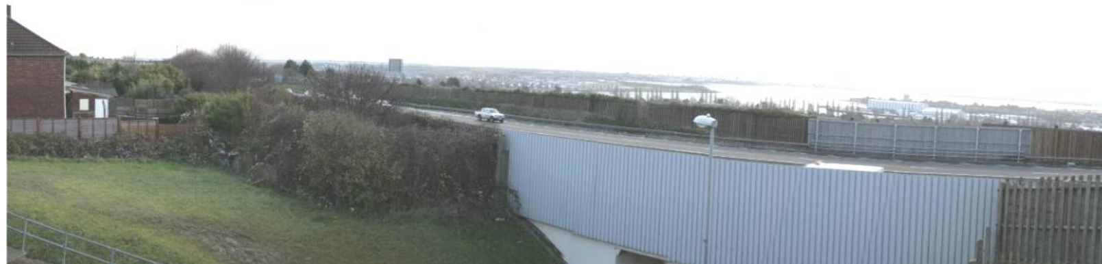
Figure D.11 – POPE OYA view looking south from Hillsley Road: View illustrates former lighting columns now removed and westbound climbing lane.
