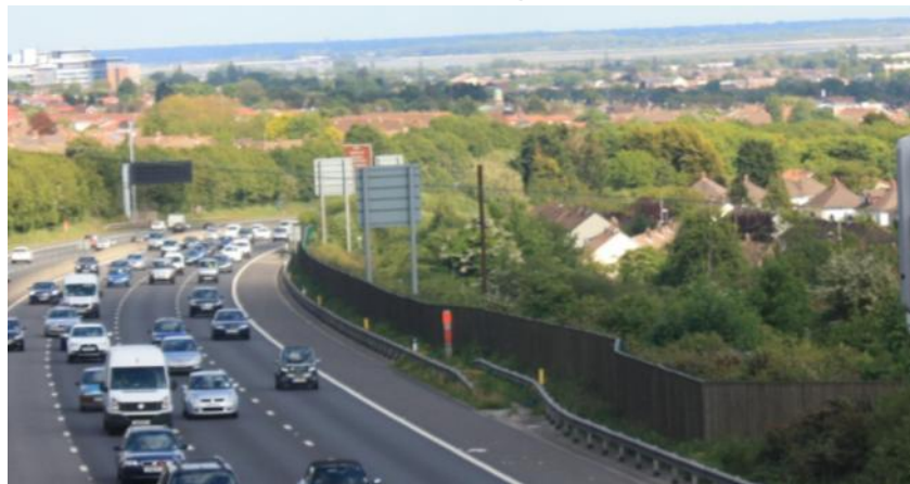
Figure 5.4 – View of acoustic barrier near Anson Grove looking east from High Tor Overbridge
