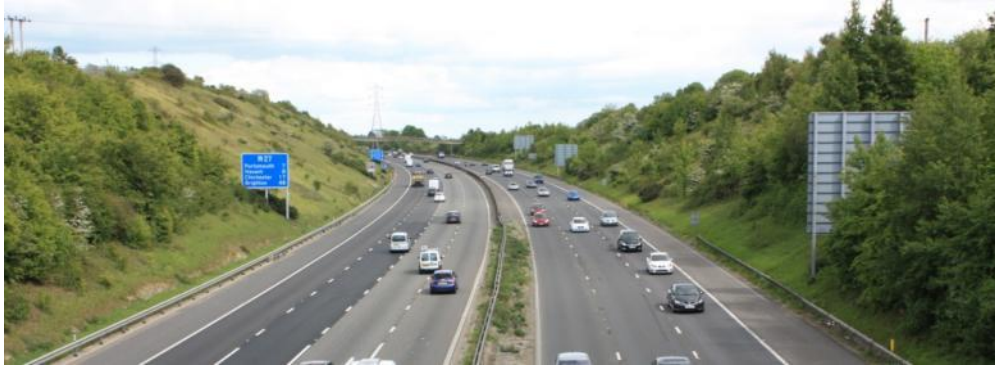
Figure 5.2 – View of the scheme looking east from the Downend Road overbridge showing the start of the eastbound climbing lane
