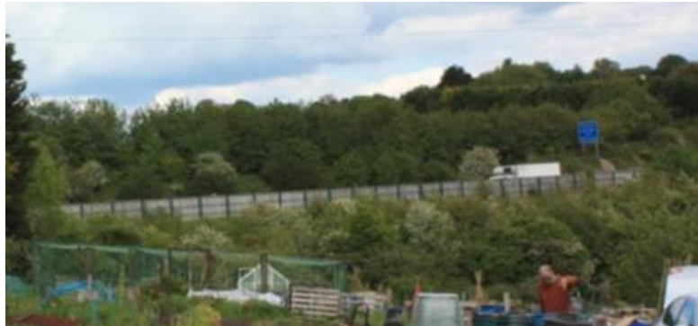
Figure 5.3 – The noise / screening barrier adjacent to the Cornway Allotment Gardens, Danes Road
