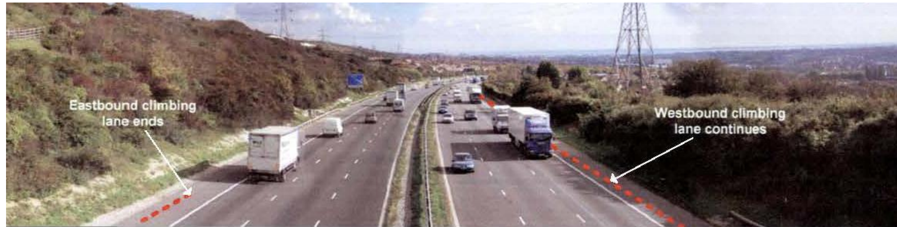
Figure D.7 – ES Figure 9. 4b – Viewpoint D: High Tor Footbridge looking east (FP119B) - summer
