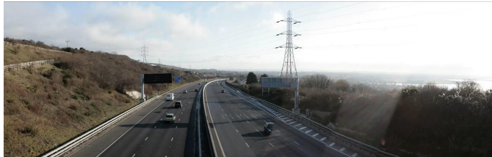
Figure D.8 – POPE OYA view looking east from High Tor footbridge: View illustrates westbound climbing lane, retained signage (eastbound carriageway) and new VMS
