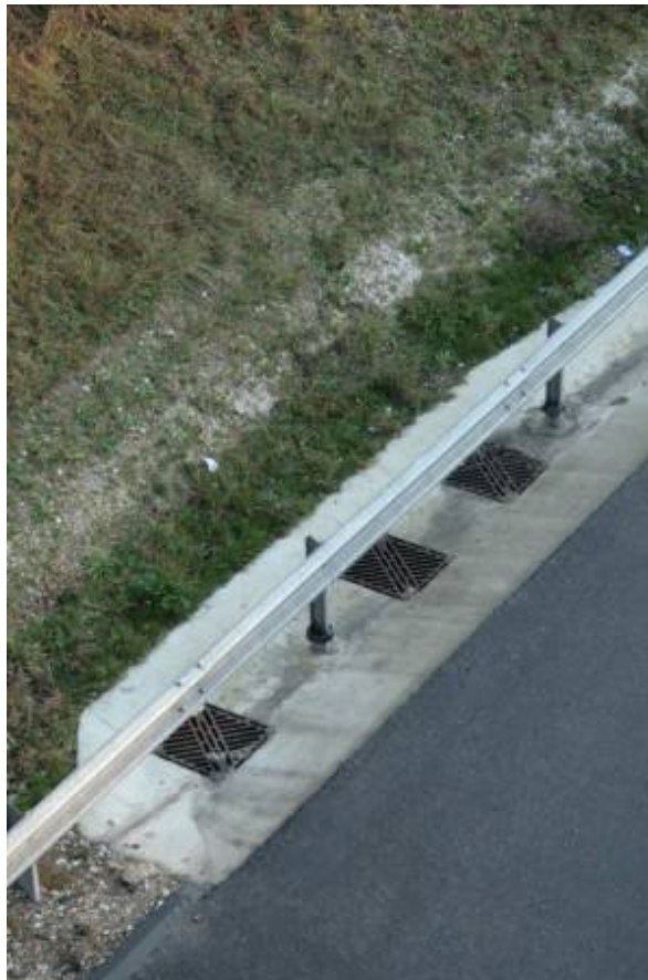
Figure 5.6 – Drainage channel and gully and restored tie in with chalk verge
