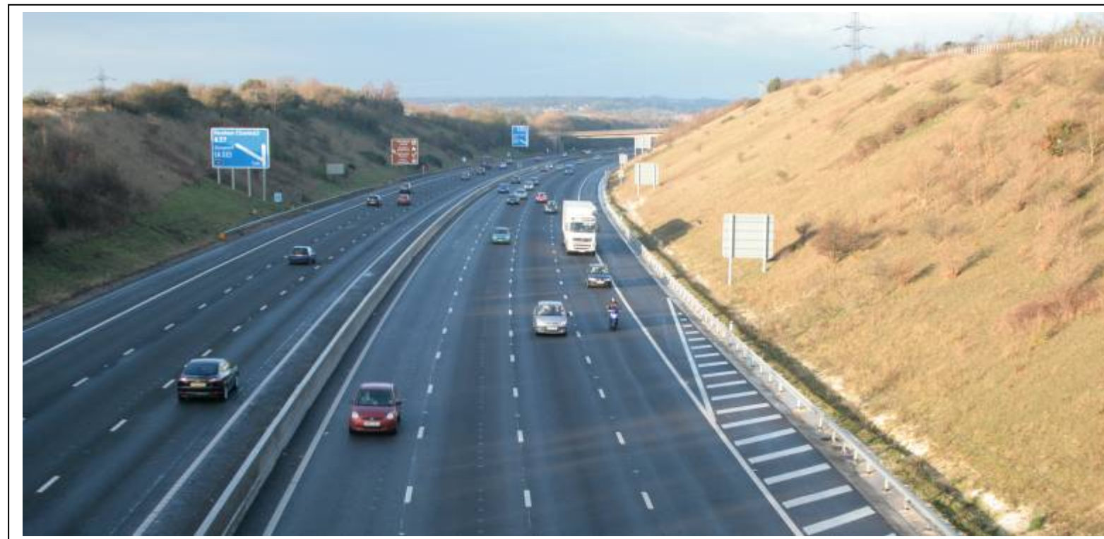
Figure B.2 – POPE view looking west from Upper Cornaway footbridge: View illustrates the deep motorway cutting, westbound climbing lane, open chalk verges and slightly amended signage layout (eastbound)
