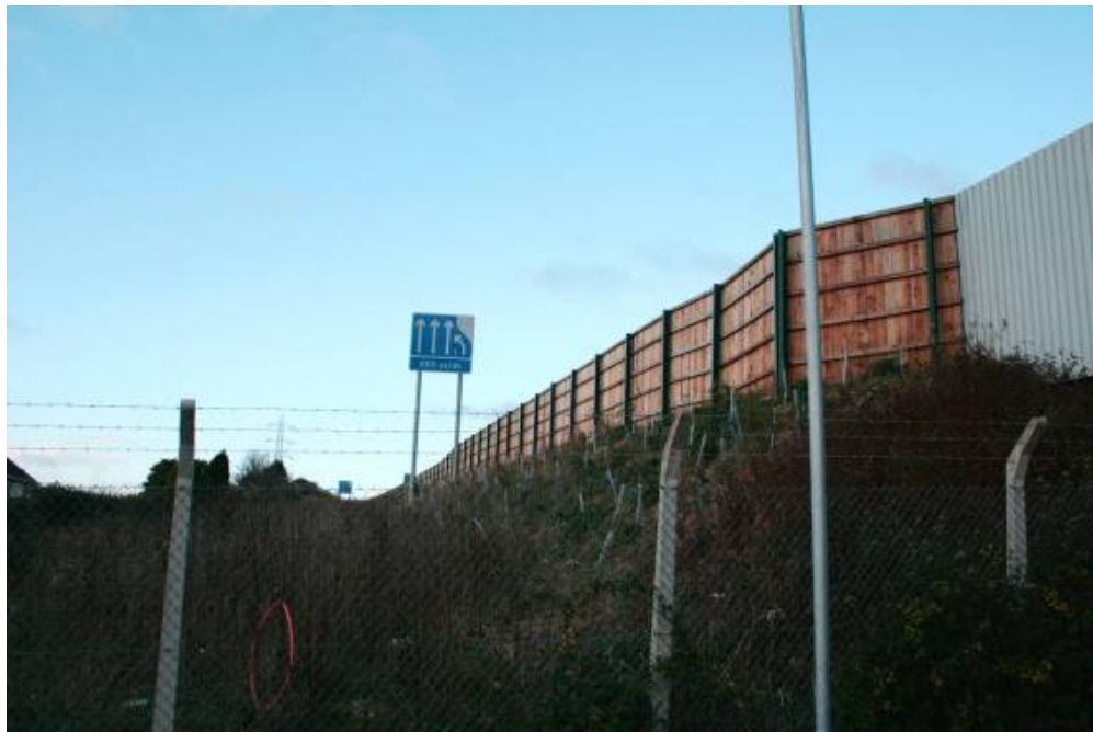
Figure 5.1 – Acoustic barrier to the north of Browning Avenue
