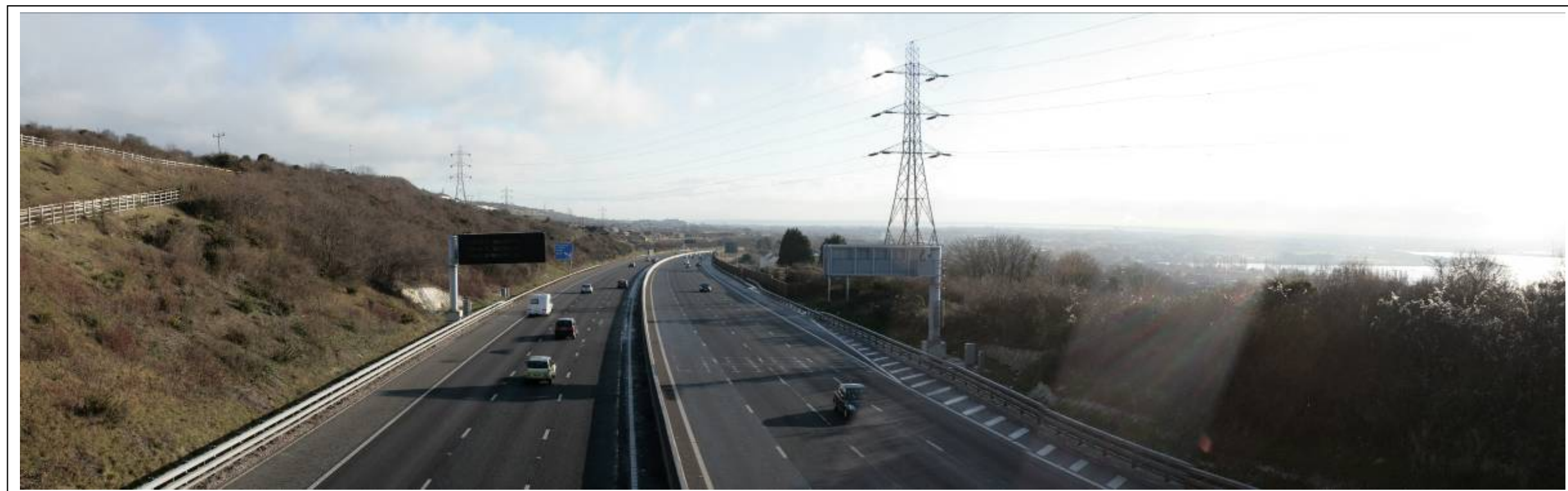
Figure B.6 – POPE view looking east from High Tor footbridge: View illustrates westbound climbing lane, retained signage (eastbound carriageway) and new VMS
