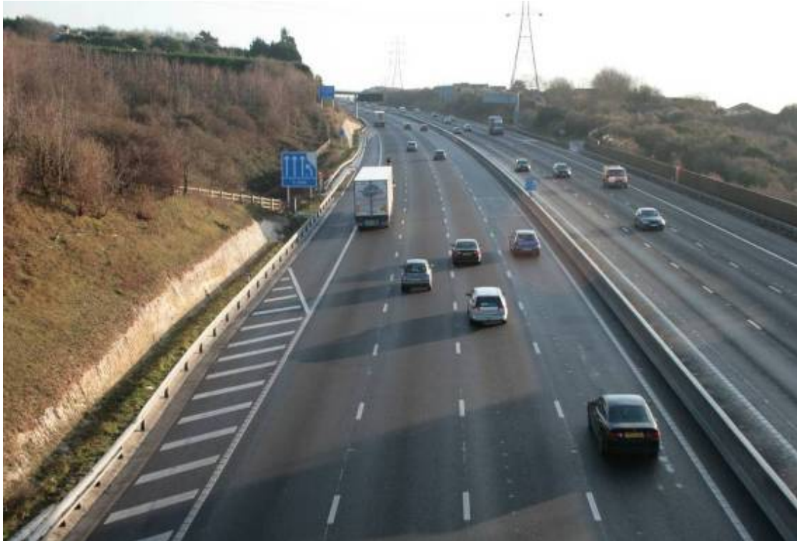
Figure 5.8 – View of the motorway corridor and the vehicle travellers experience looking east from Upper Cornaway Lane footbridge
