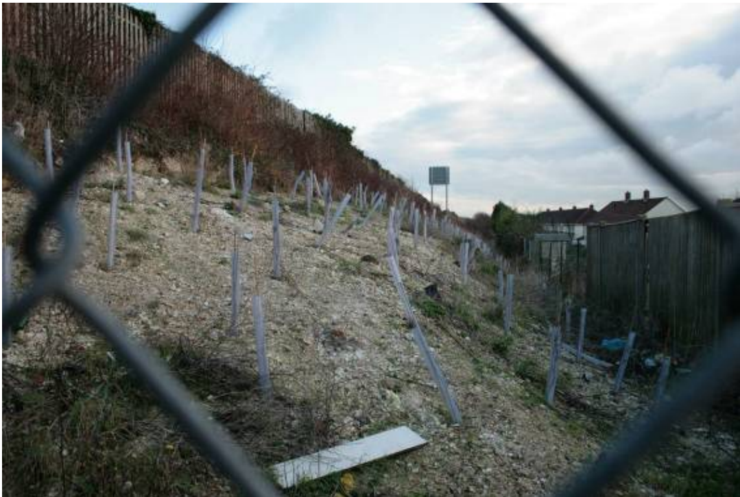
Figure 5.2 – Small scale landscape mitigation planting at Hillsley Road Subway
