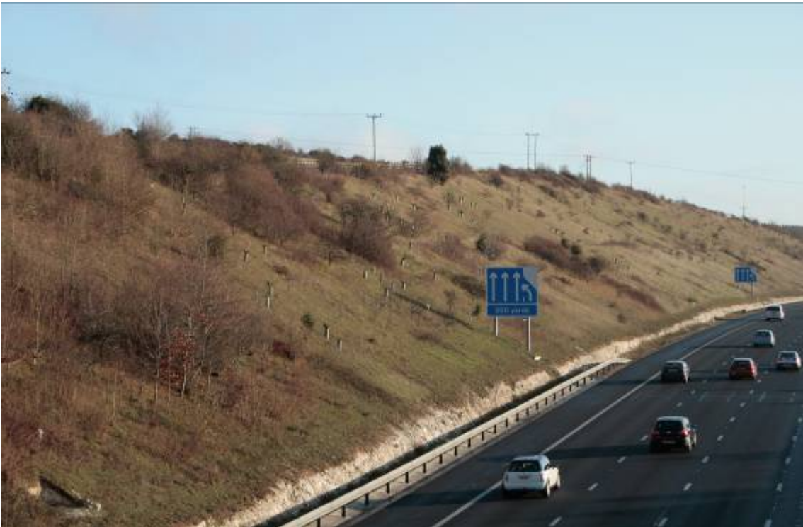
Figure 5.5 – Typical example of retained habitat and vegetation cover
