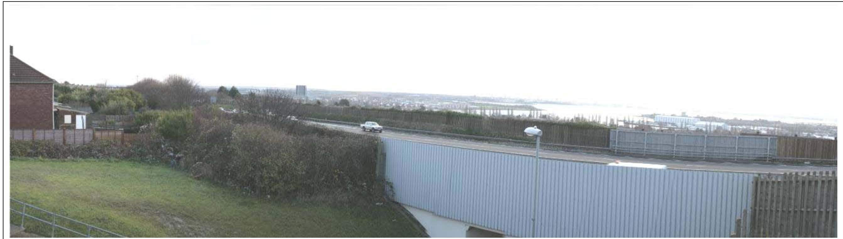
Figure B.8 – POPE view looking south from Hillsley Road: View illustrates former lighting columns now removed and westbound climbing lane.
