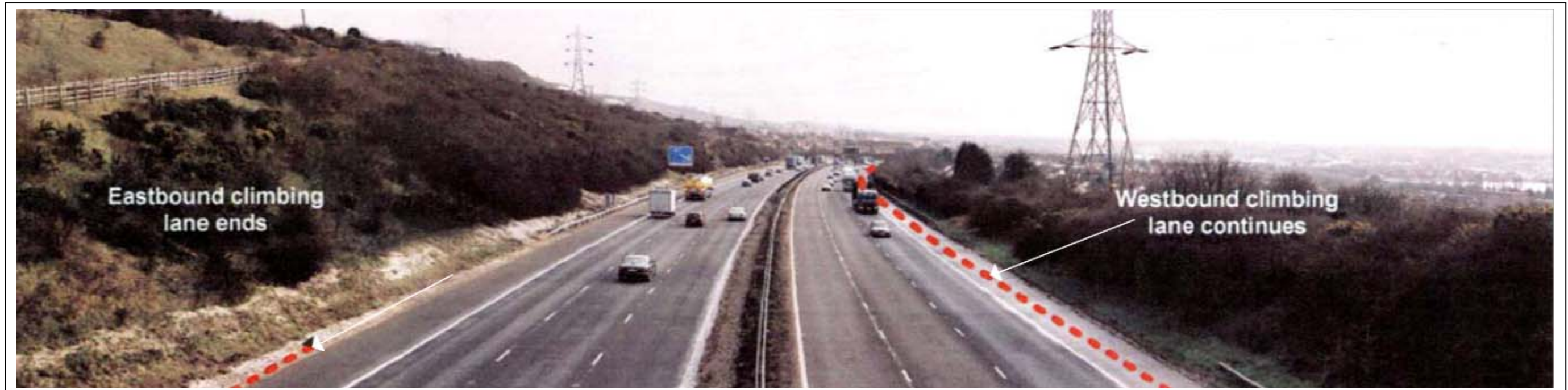
Figure B.5 - ES Figure 9. 4b – Viewpoint D: High Tor Footbridge looking east (FP119B) - Winter
