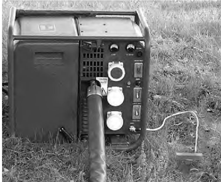
Fig 1 Earth spike and LFG earth terminal
