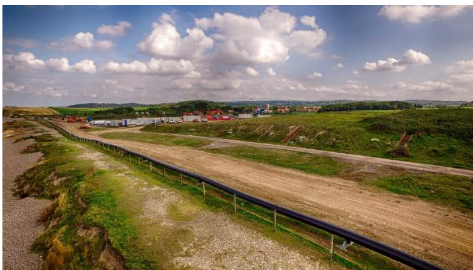
Laid cable – surface
