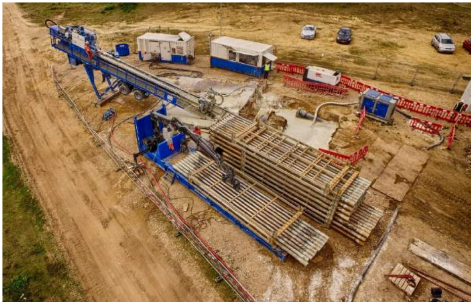
Rig set up and HDD site
