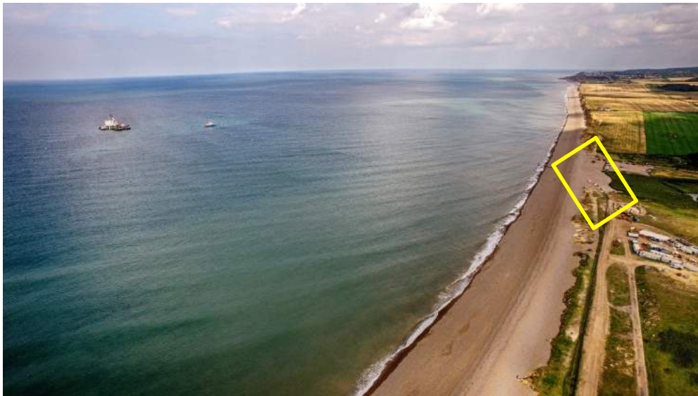
Landfall and HDD site
