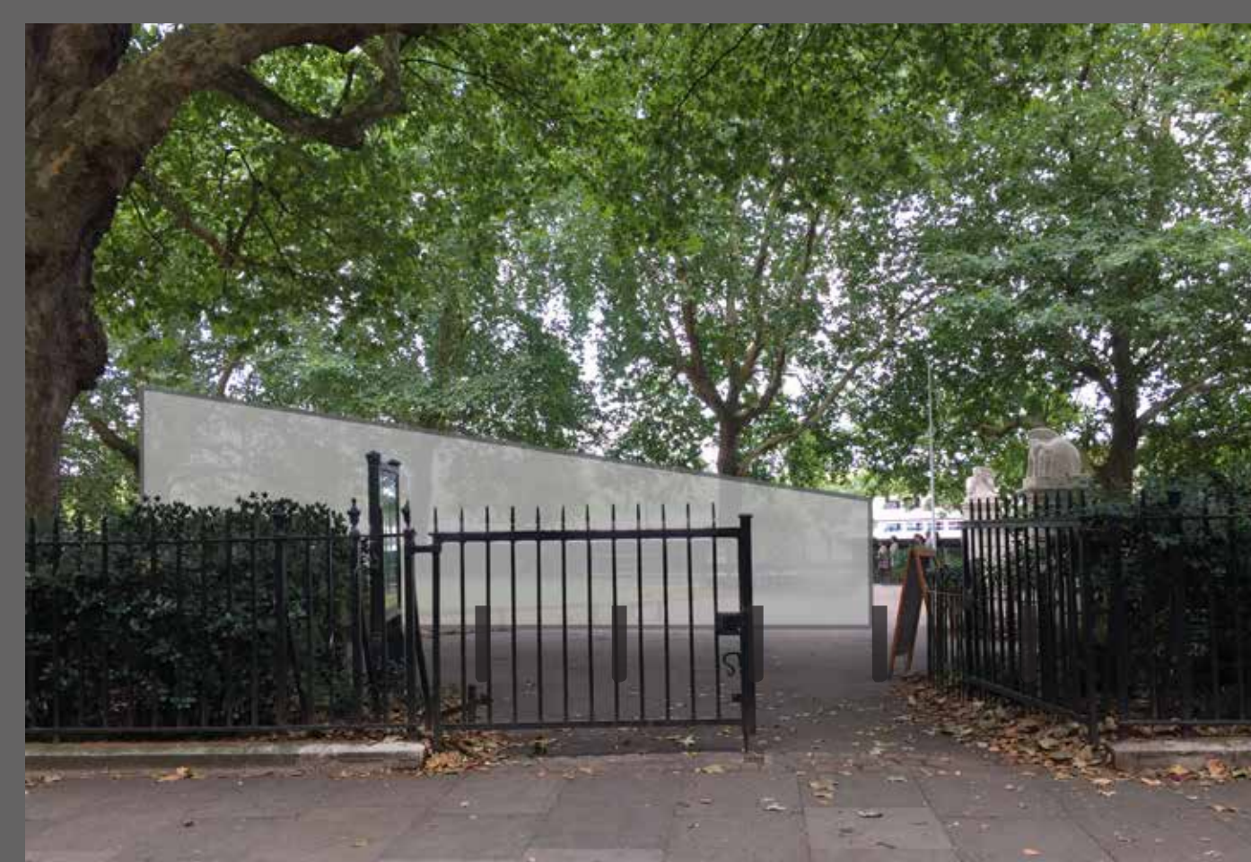
Entrance 4: showing Entrance Pavilion on Millbank
