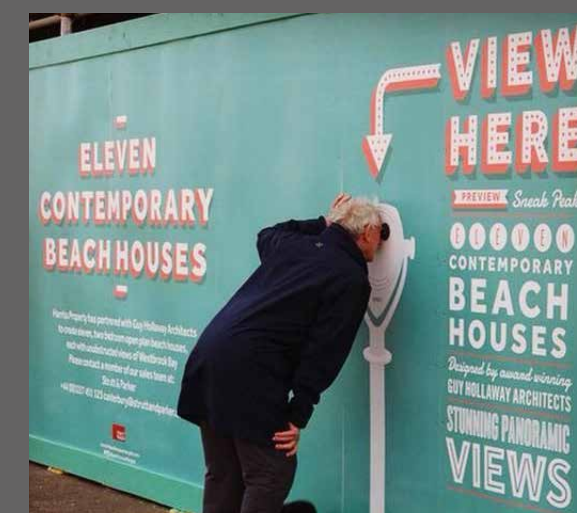
Viewing window in hoarding example © Brett Pierson
