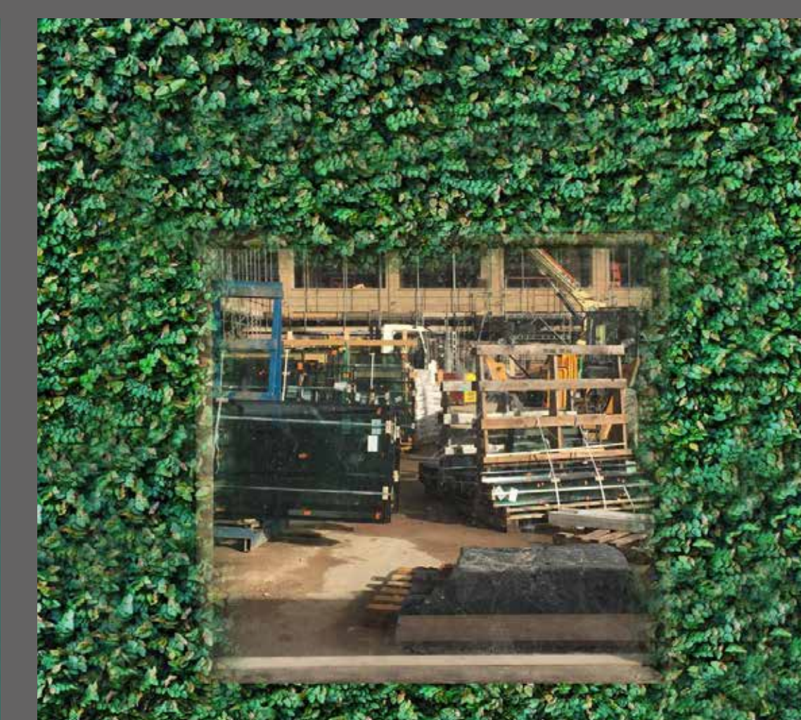
Viewing window in hoarding example © Worcester University
