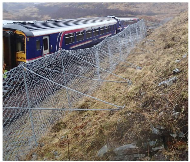
Figure 15: Detailed view of catch-fence supported by anchored cables
