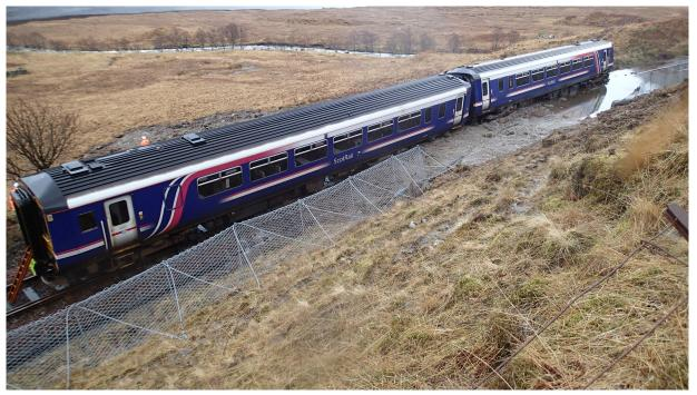
*Figure 14: Part of catch-fence installed in 2017 to trap falling rocks and boulders. The middle section was destroyed by the landslip. Part of the railway boundary fence is also visible in the foreground.*
