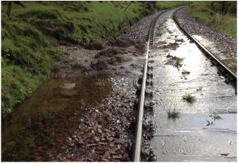
Figure 13: view of minor landslip which occurred in June 2015 about 150 metres west of the 2018 accident landslip (photograph courtesy of Network Rail)
