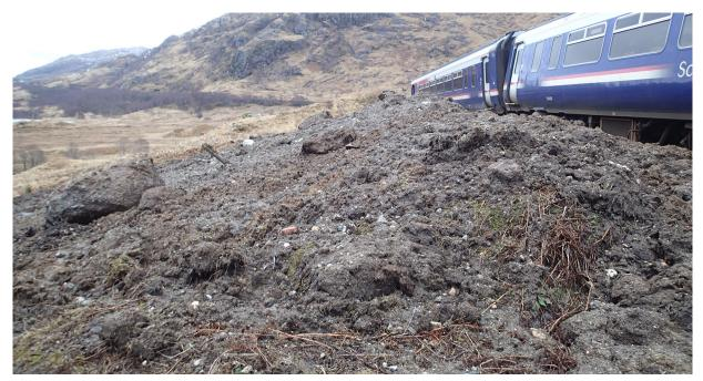
Figure 11: View showing nature of debris on downhill side of railway
