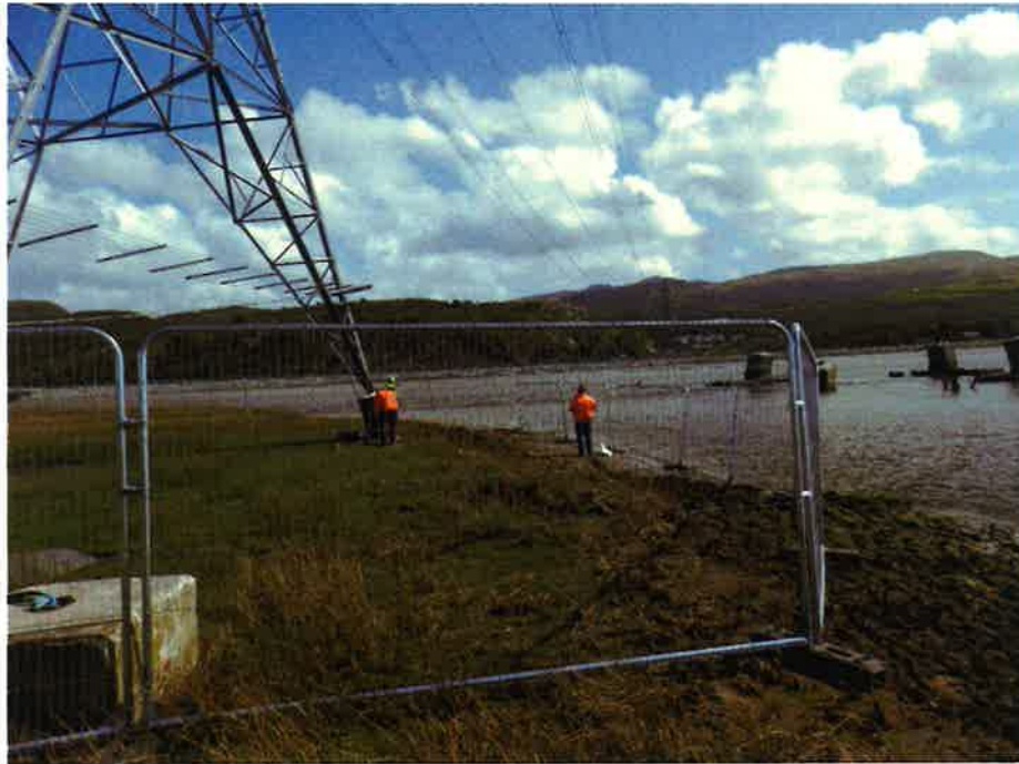
Figure 7. Saltmarsh and Tower 4ZC030T prior to commencement of cofferdam installation
