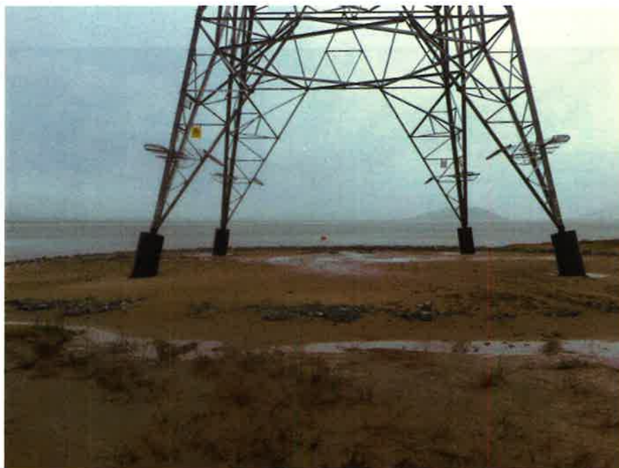
Figure 9. Tower 4ZC030T and cofferdam, immediately following installation
