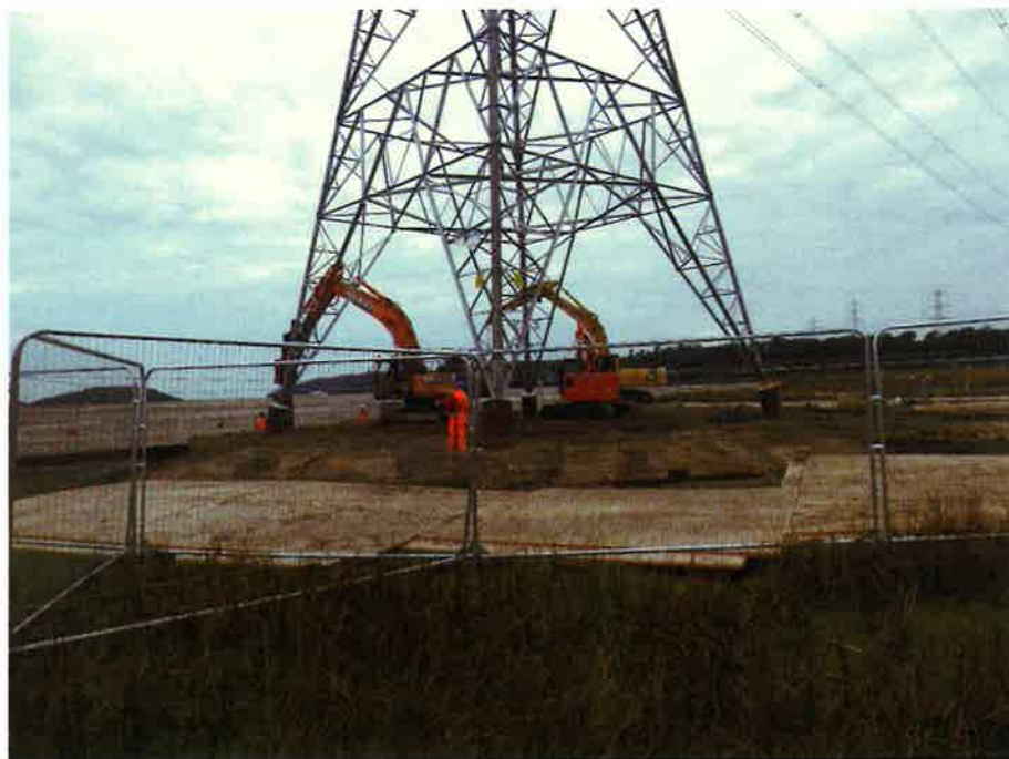
Figure 8. During coffer dam installation
