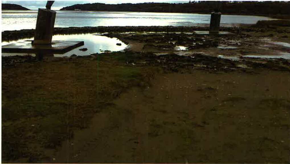
Figure 4. Scour and saltmarsh habitat within cofferdam, looking west
