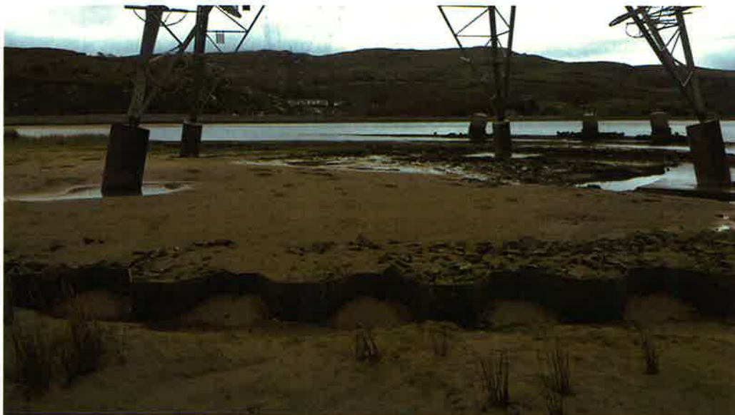
Figure 1. Habitats within cofferdam of 4ZC030T looking southeast
