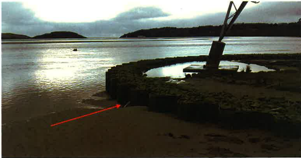
Figure 6. View of water draining from the cofferdam (see arrow)
