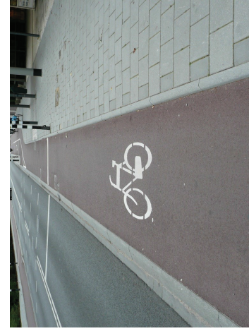
Danish style 'stepped track', providing a less formal approach to segregated cycle tracks.
