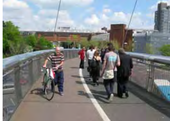
33 New shared use bridge over railway at Aylesbury Station
