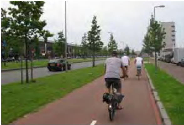
9 Cycle track set well back from main road and separated by avenue trees. (Rotterdam)
