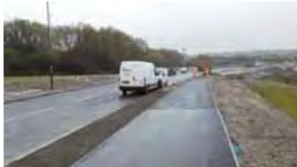
59 New link road to Woodthorpe
