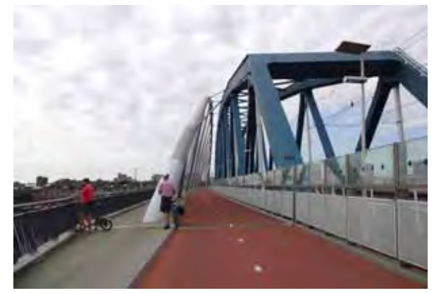
35 Major new cycle route attached to railway bridge approaching Nijmegen
