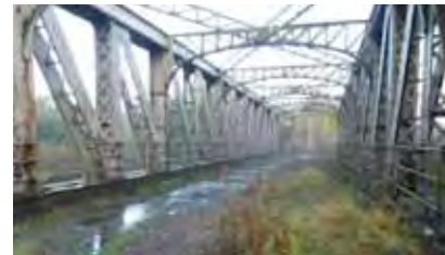
43 Remaining bridge over the River Don
