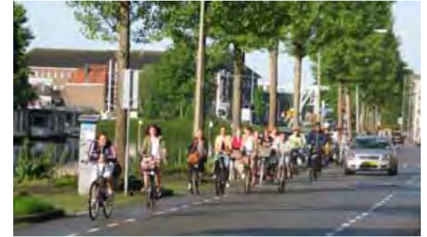
6 Where space is limited the removal of the central white line and introduction of advisory cycle provision emphasises the presence of cyclists. (Gouda)
