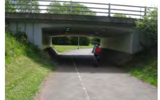
36 Wide, on the level, underbridge at Tamworth
