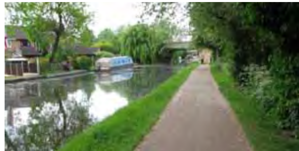
14 Narrow 2m wide towpath on Erewash Canal; note sealed surface with appropriate coloured gravel
