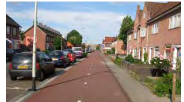
8 Reallocation of road space through residential development to create 2 way cycle route. (Breda)
