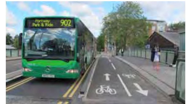
7 One lane of the road made into a two way cycling track (Redcliffe Bridge, Bristol)
