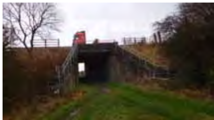
48 Bridge under M1 leading down to Rother Valley Park
