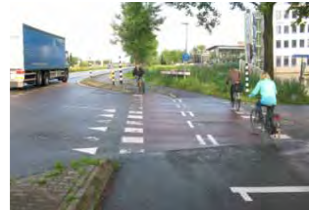
27 Path continuing parallel to main road (Gouda). Note the crossing is arranged on the desire line
