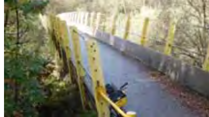
36 TPT bridge over River Dearne
