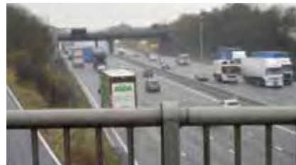
52 M1 at Barlborough
