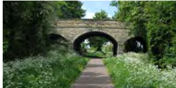
12 Typical railway path, 2.5m wide rural areas, 3.0m minimum urban areas. (Derby, Melbourne)
