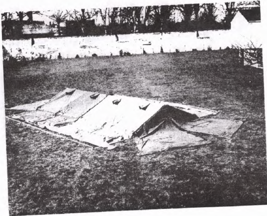
Fig 19 - Lace covers together as shown in Figs 5 and 6. Lay the covers over the assembled roof frame and fit bracket ends into the sleeves provided on the end.
