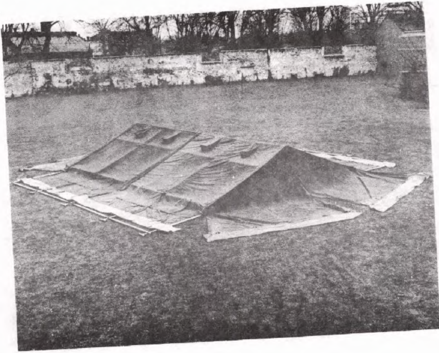
Fig 9 - Lay the three shelter lashings over the cover as shown.
