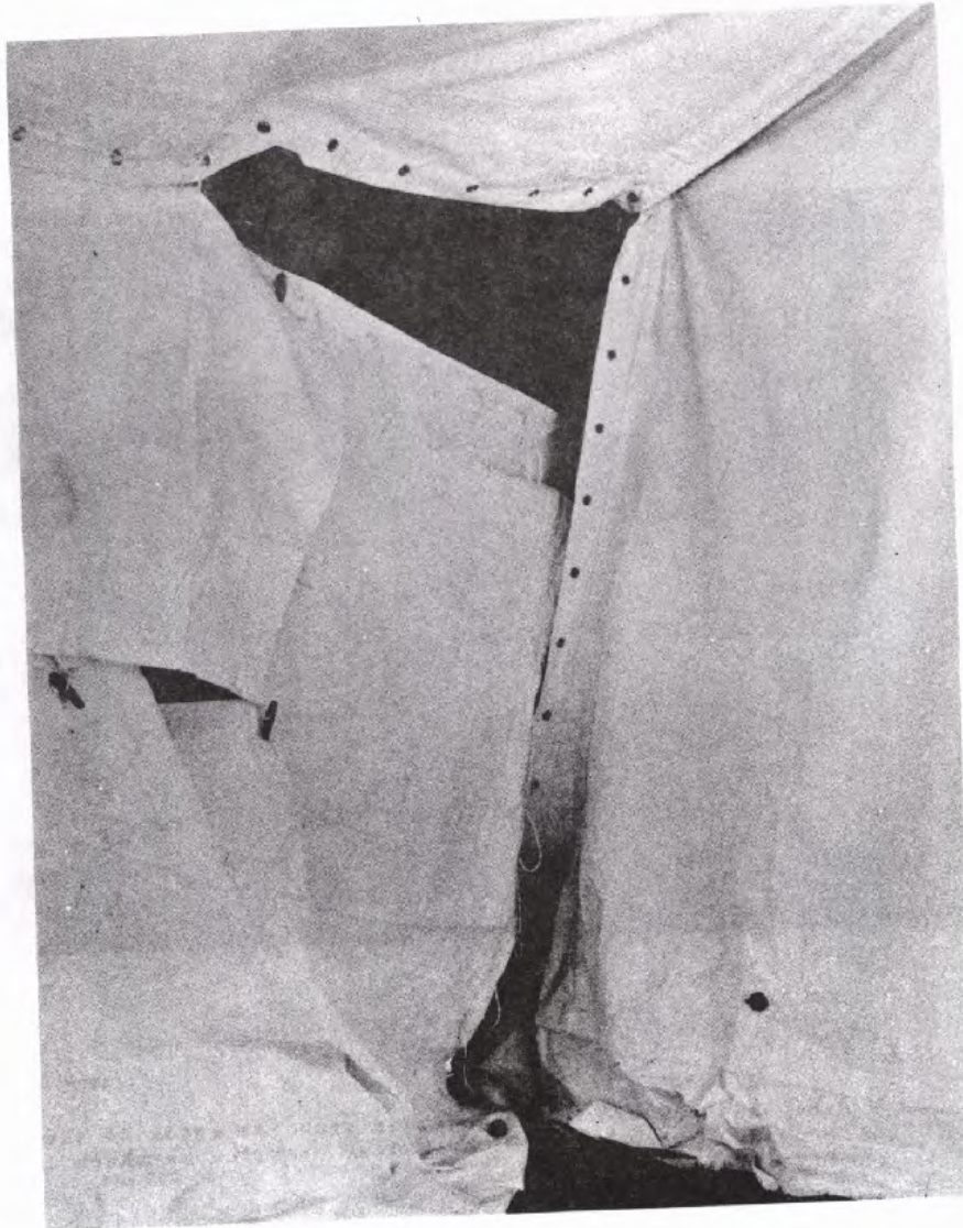
Fig 23 - Follow erection instructions shown in Figs 4 to 11. After stage 11 fit liner walls by lacing the walls to the eaves of the roof.
