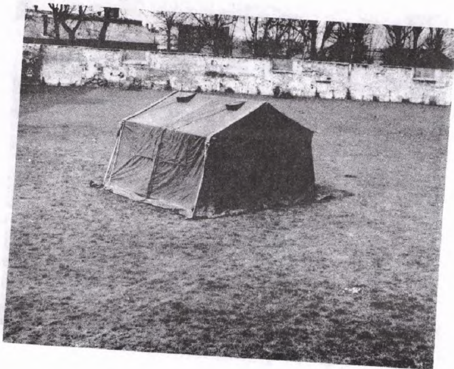
Fig 10 - Raise the other side of the roof and fit wall and ground members
