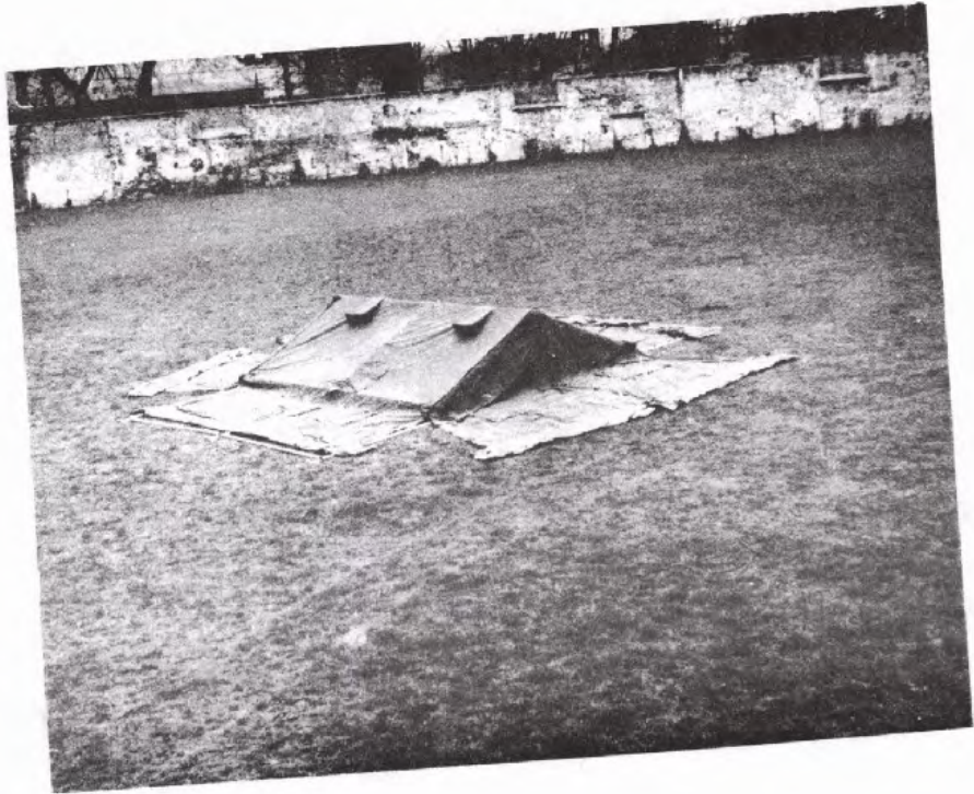
Fig 7 - Lay cover over the assembled roof and fit bracket ends into the sleeves provided on the end covers.
