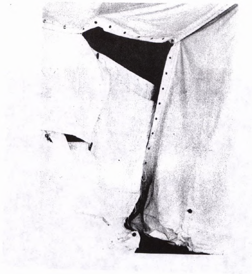
Fig 26 - Follow erection instructions shown in Figs 3 to 10. After stage 10 fit liner walls by lacing the walls to the eaves of the roof.
