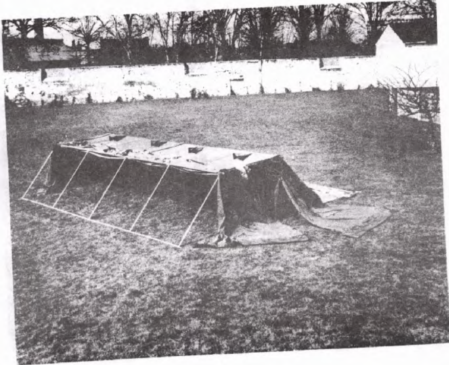
Fig 21 - Raise one side of the roof and fit wall and ground members. One man is required for each wall member and the lift must be even to avoid damage to the frame.
