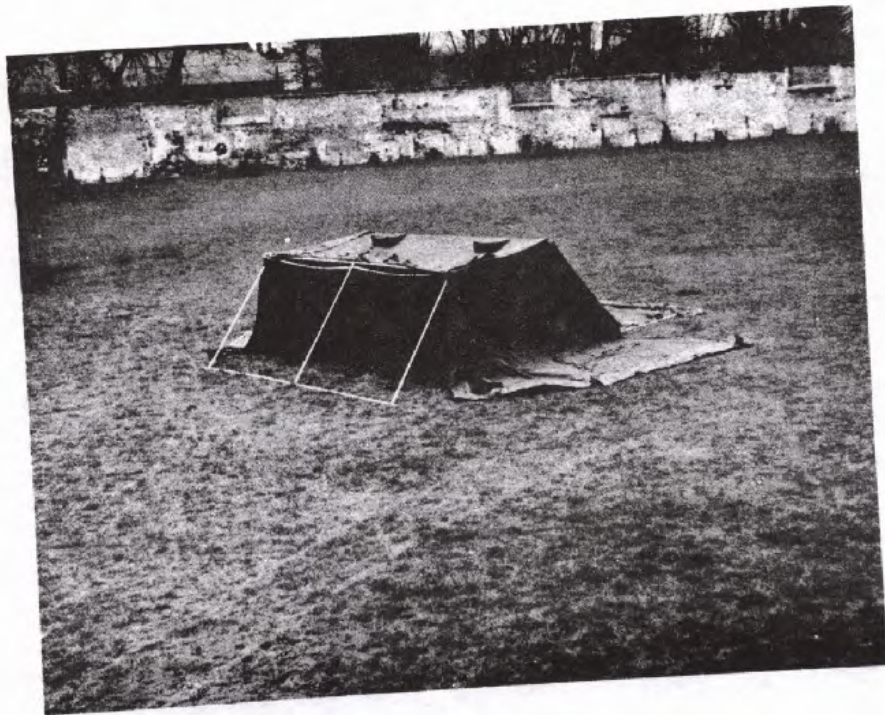
Fig 9 - Raise one side of the roof and fit wall and ground members. One man is required for each wall member and the lift must be even to avoid damage to the frame.
