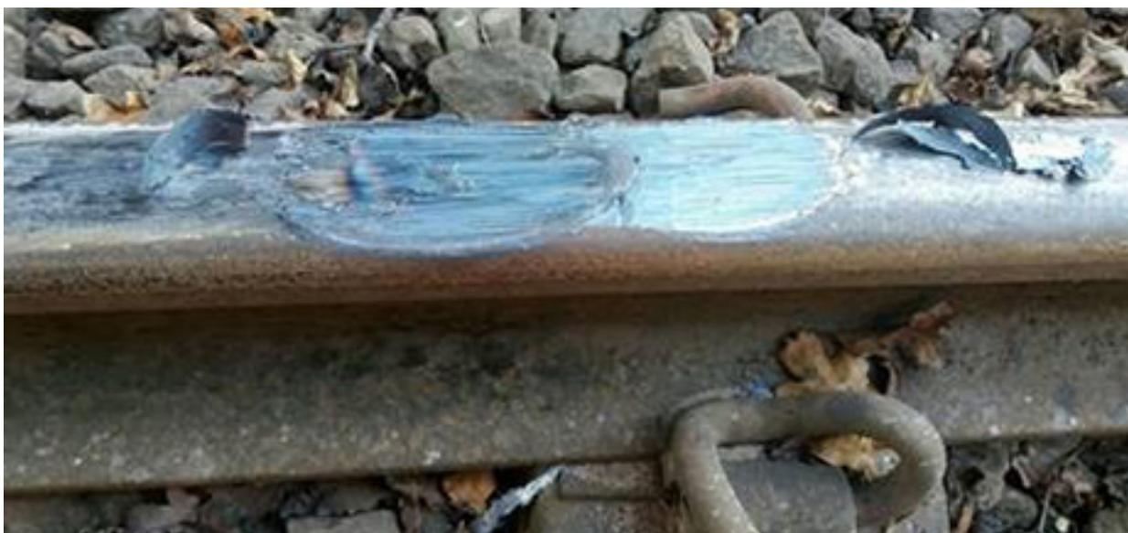
Figure 7: Damage to the rail head 67.2 miles (108.1 km) from Roboston (courtesy Network Rail)
