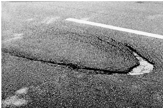
Cracking outside wheeltracks – parabolic crack
