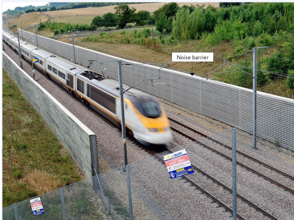
Figure 22: Photograph of a noise fence barrier
