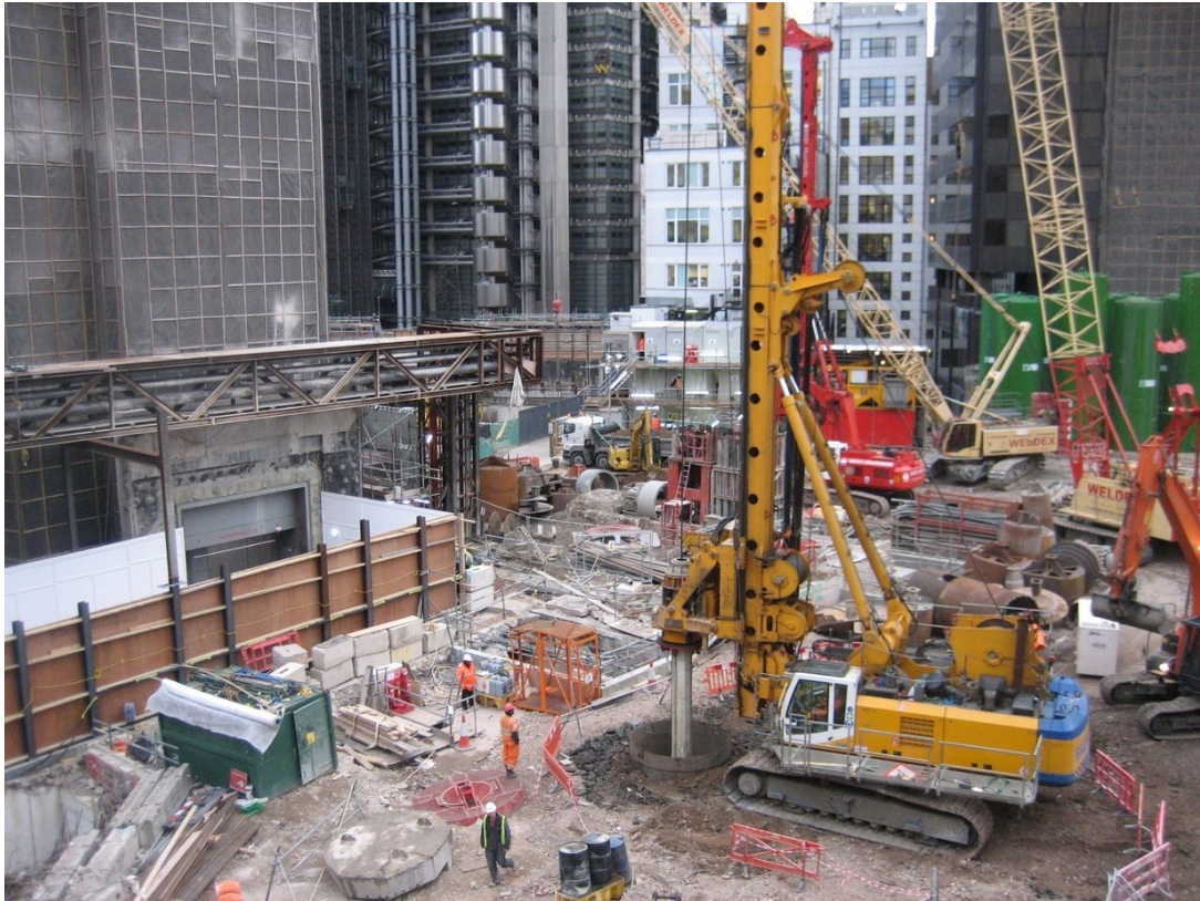
Figure 29: Photograph of an example of a piling rig
