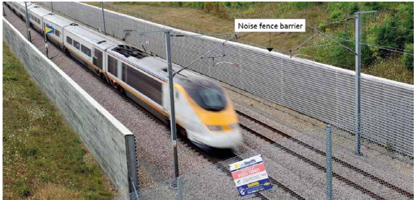
Figure 13: An example of a noise fence barrier
