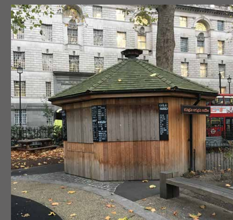
Kiosk to be replaced with renewed cafe area. Image courtesy of Adjaye Associates
