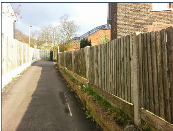
Ladbroke Road Alleyway - New tarmac surface constructed to replace previous mud surface. This is one of the few options for pedestrians to cross the railway, and avoids the need for a lengthy diversion into the town centre, to cross at the station.
