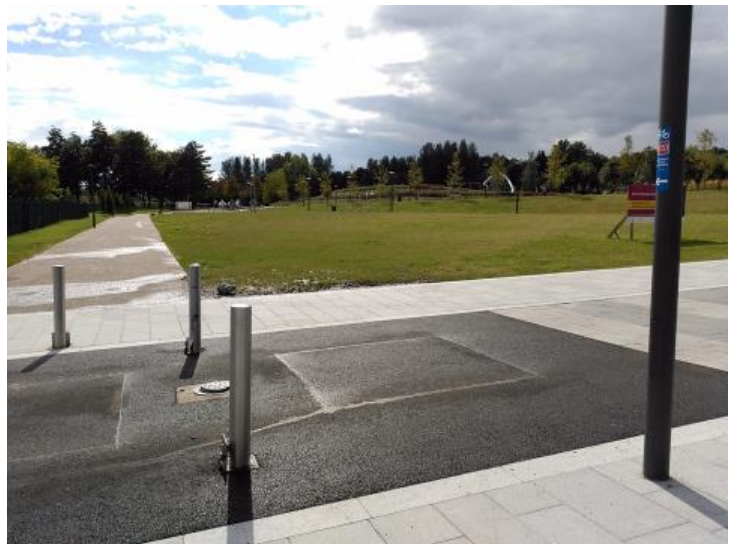
Post LSTF investment (August 2015). Toucan Crossing at Telford International Conference Centre.
