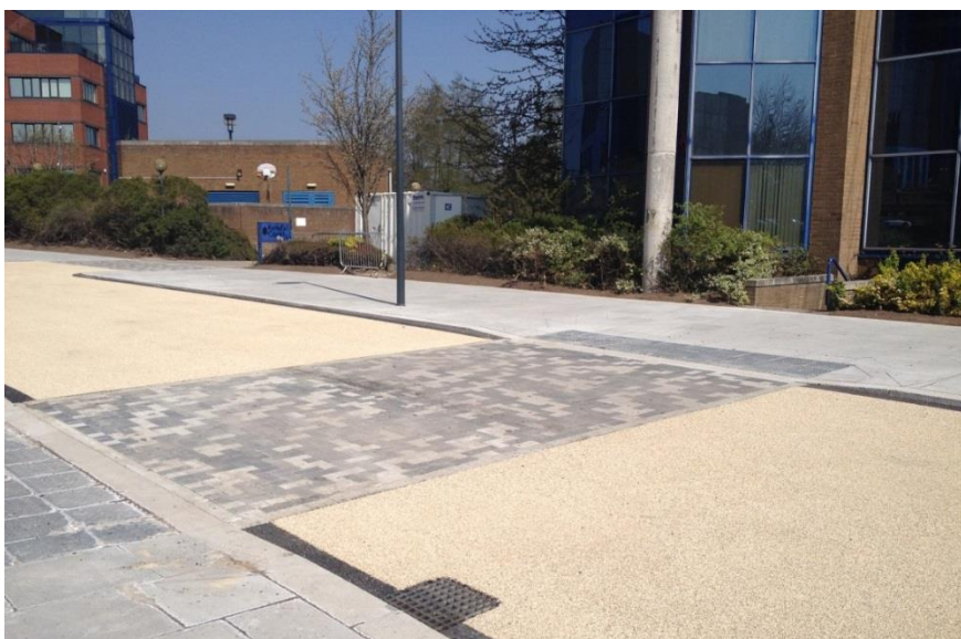
Post LSTF investment (April 2015). Application of shared space principles on Ironmasters Way – low kerbs and level courtesy crossing.
