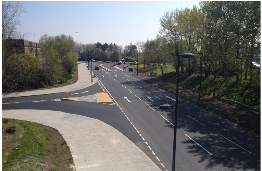
Looking east along Lawn Central towards Grange Central
