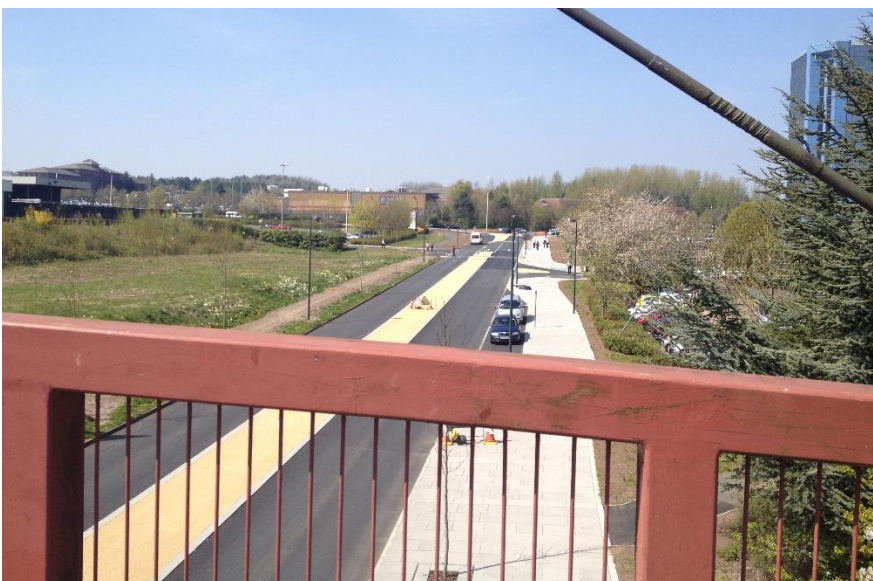
Looking west along Lawn Central towards Woodhouse Central – Highway capacity reduced from three to two lanes. Wide central reservation provided to make it easier to cross. Shared space principles in terms of low kerbs and courtesy crossings not applied on Lawn Central due to volume of traffic. Wide shared cycle / footways provided adjacent to traffic on outside of Box Road. New lighting.
