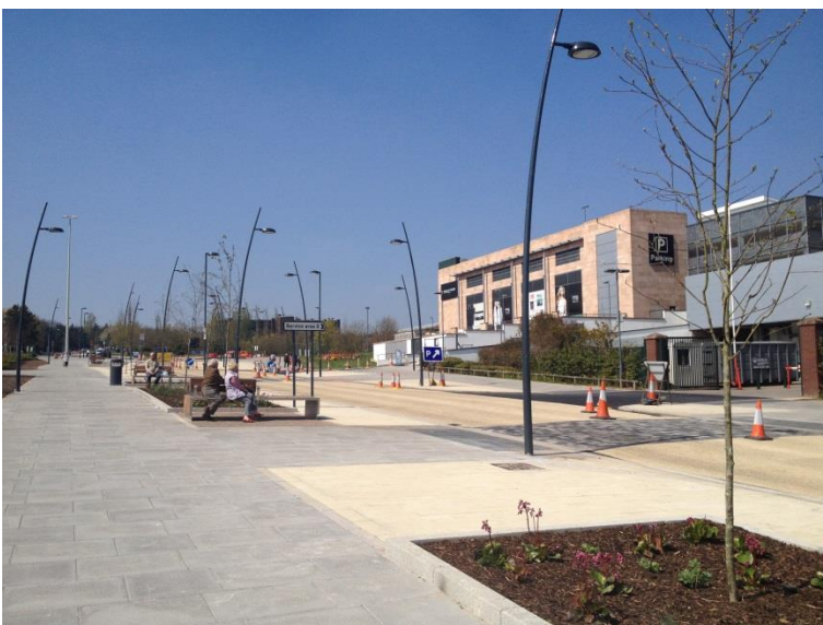
Coach Central - Looking north west along Coach Central towards Woodhouse Central – Shared space with courtesy crossings; new lighting, street furniture and landscaping.
