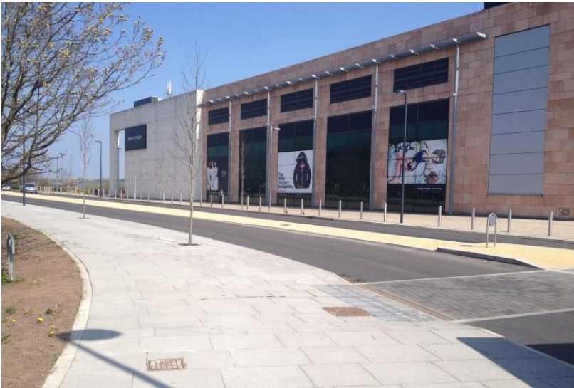
Figure 7. Woodhouse Central – After LSTF investment (April 2015)
