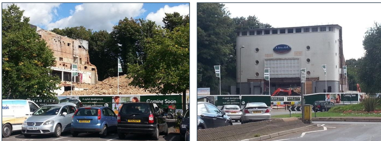
Figure 36. Station Road Redevelopment (Photo - August 2014)
