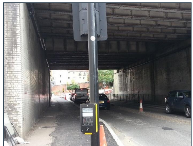
Poor quality pedestrian environment under the Railway Bridge on Station Road
