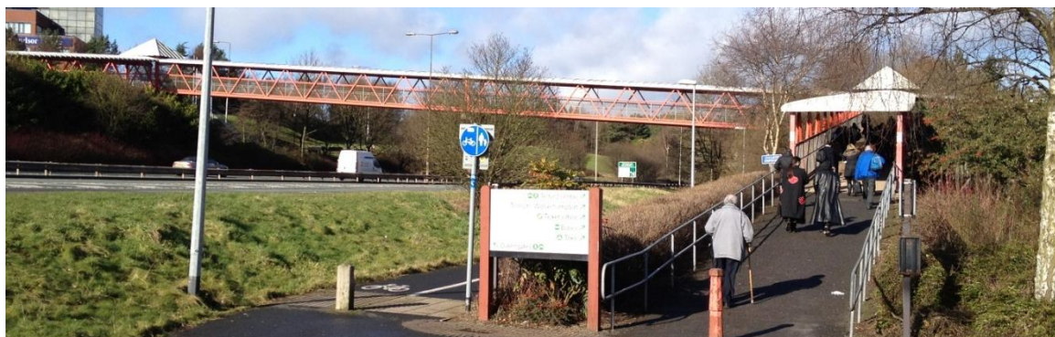
Figure 12. A442 / A5 pedestrian and cycle overbridge from rail station (existing)
