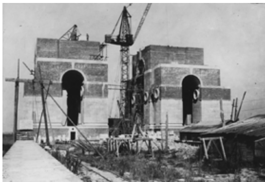
The Thiepval Memorial under construction © CWGC
