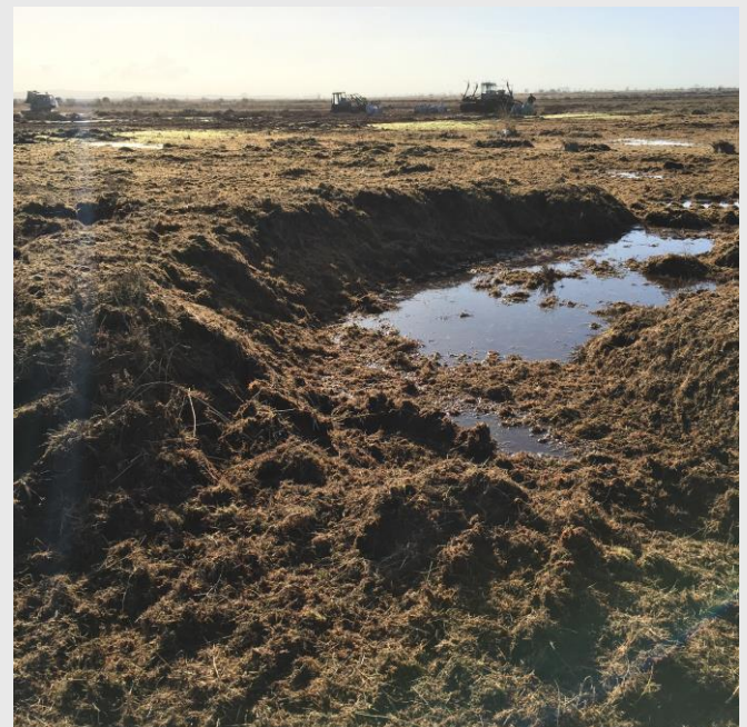
One of the bunds holding water on the bog surface, which has recently been re-vegetated with the sphagnum/heather/grass mix.
