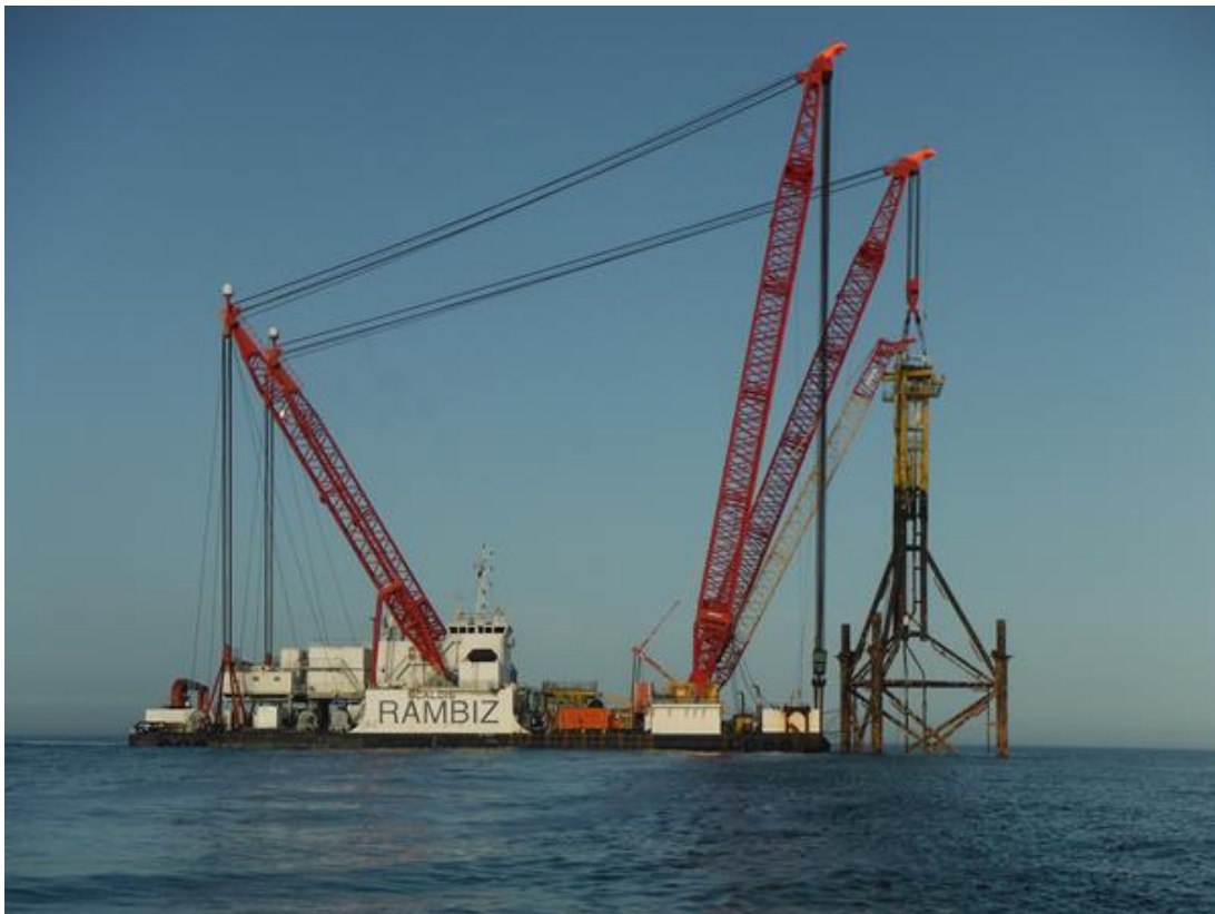
Figure 4.4 Rambiz 3000 HLV having lifted Horne & Wren Platform
