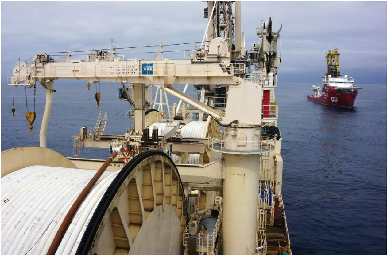
**Figure 9 : Edradour Flowline Installation**
