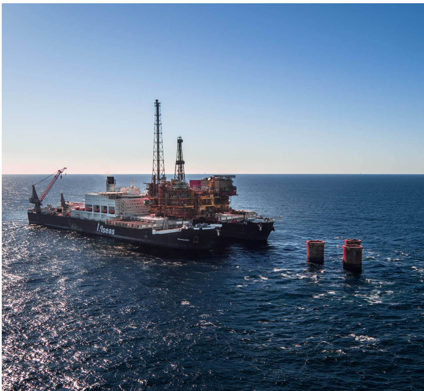
Brent Delta Topside removal by Pioneering Spirit , April 2017.
