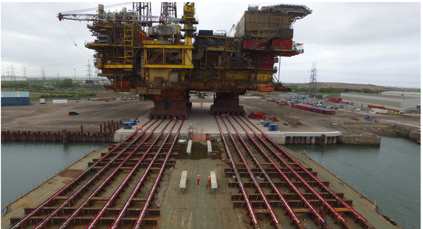
Brent Delta Topside Skidded onto Quay 6 ASP Facility Teesside, May 2017
