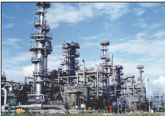
Photo 5 - POA Gas Terminal
