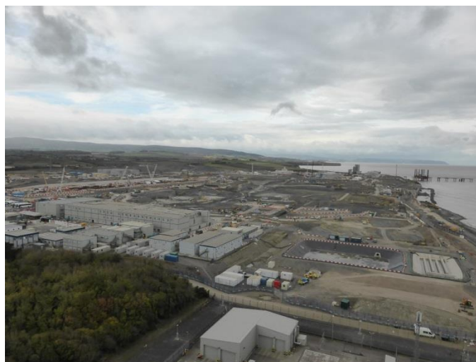
HPC Site Construction
