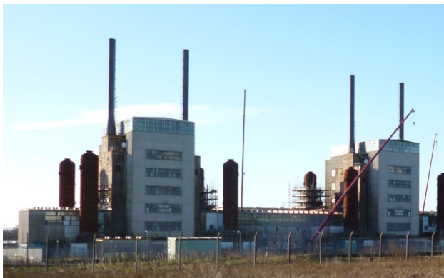
Figure 6: Reactors with top ducts removed. Steelwork and pipe work strip progressing.
