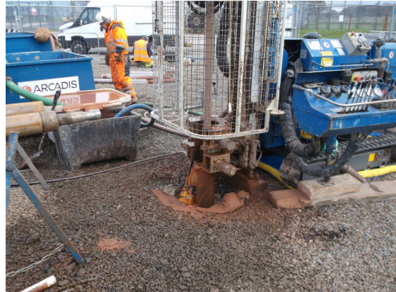
Figure 8: Solvent plume remediation works
