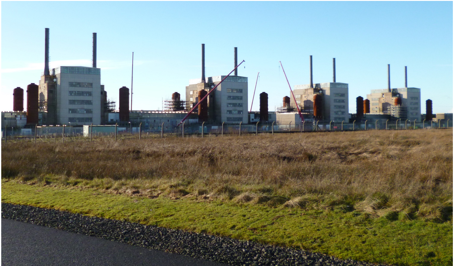
Figure 4. The Chapelcross reactors are now in the Care and Maintenance Preparations phase
