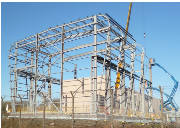
Figure 7: Construction of Intermediate Level Waste Interim Storage Facility
