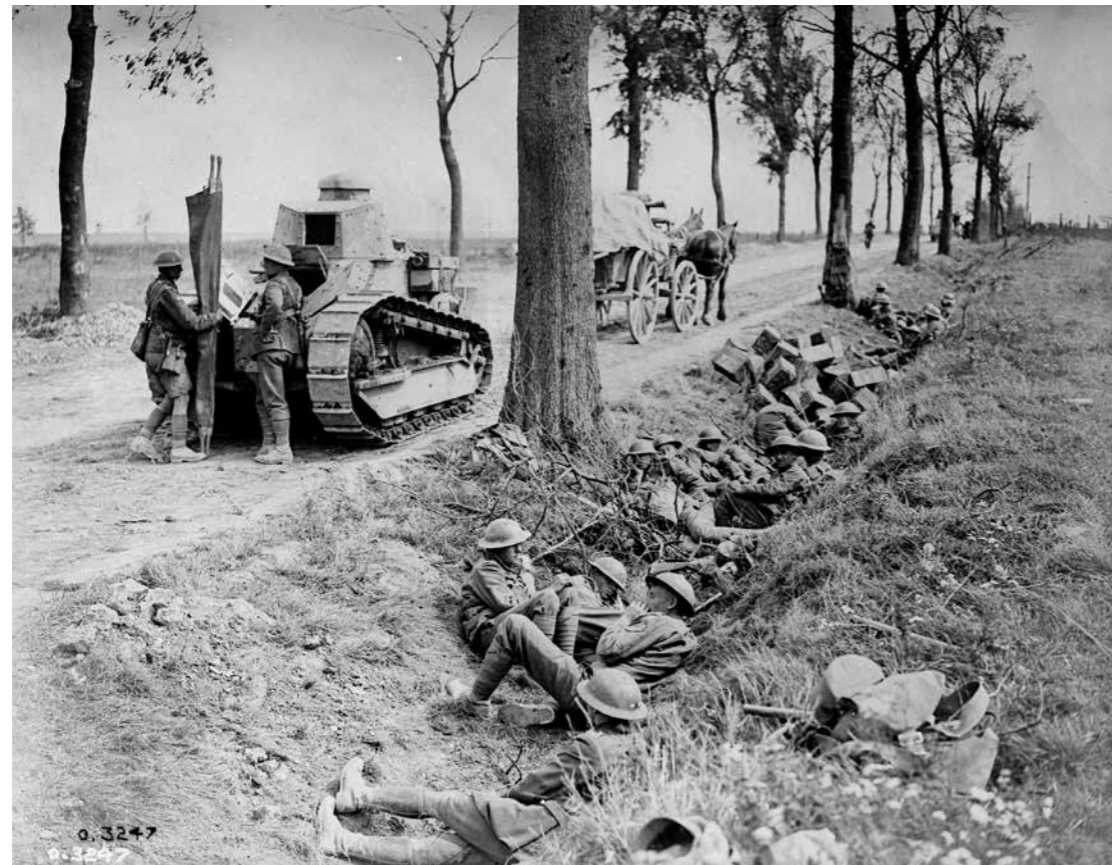
Canadian troops taking cover in a ditch alongside the road from Arras to Cambrai in September 1918. Photo: Library and Archives Canada PA-003153
