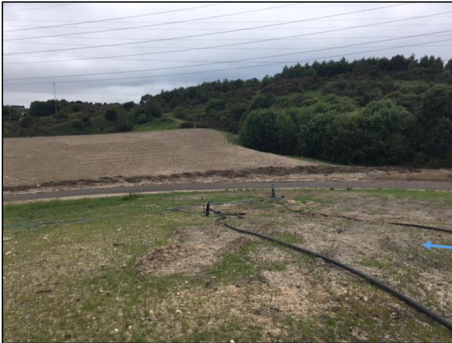
Completed area of cell 3 – looking north towards the mound.
