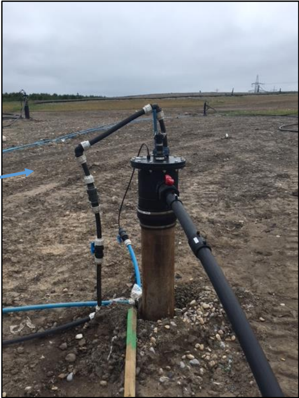
Completed gas well (steel construction) in cell 3
