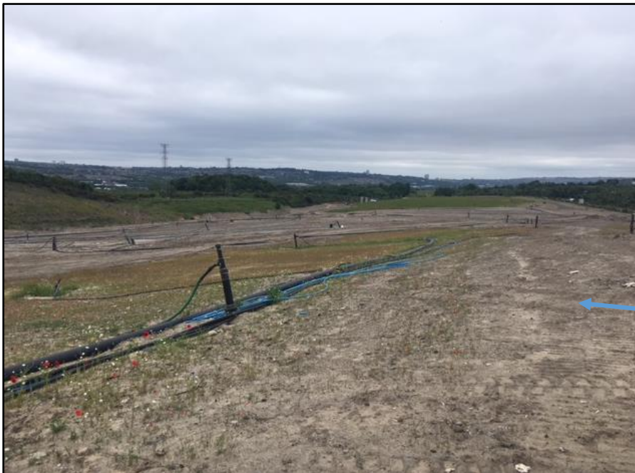
Completed area of cell 3 – looking east towards site entrance
